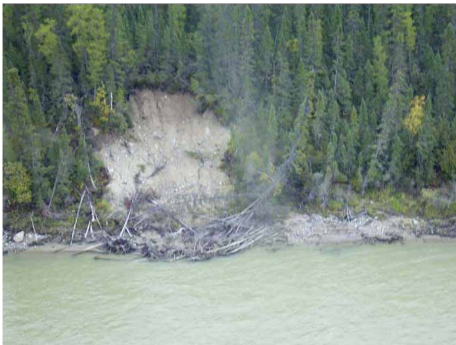
Photo 10.3-3: Localized Slope Failure in Mineral Soil Bank Between Clark Lake and Birthday Rapids. Photo Taken 19 September 2007
