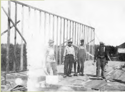
Building the Church at York Factory, 1933.
