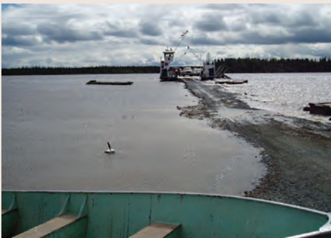
Ferry landing under high water.
