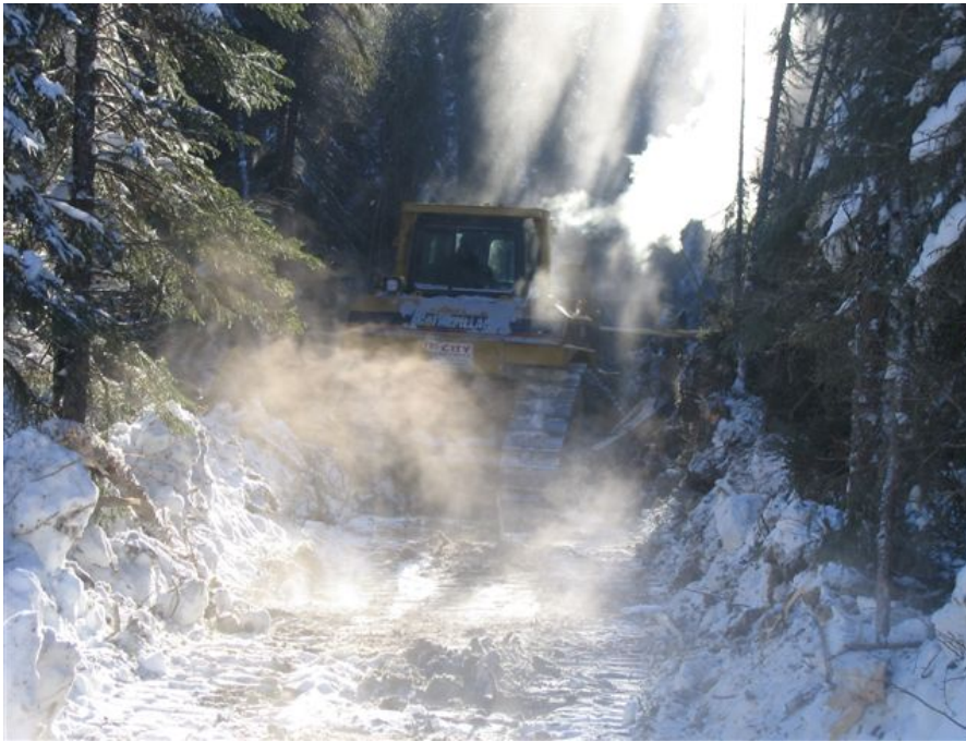
Figure 1. Clearing of vegetation using a bulldozer.
