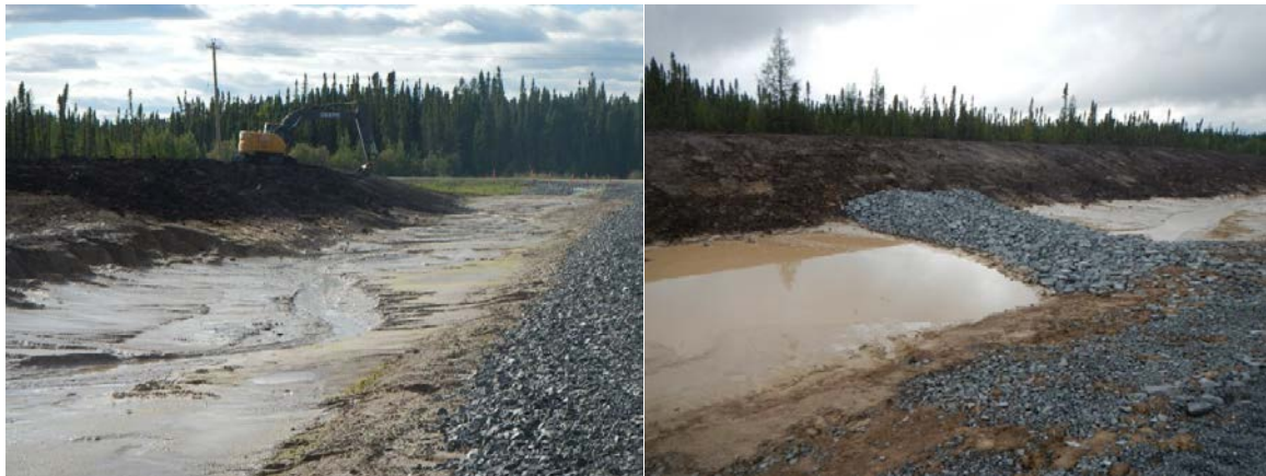
Figure 4. The access road before and after the placement of rock ditch checks.
