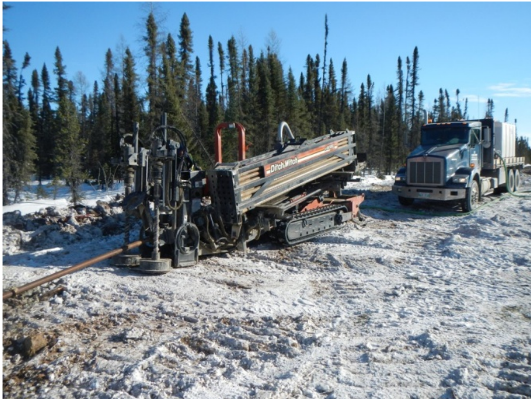
Figure 6. Machinery used in the directional drilling of the fibre optic cables at Looking Back Creek.
