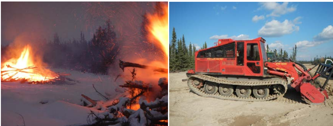
Figure 2. Disposal of cleared vegetation using burning (left) and mulching (right) methods.
