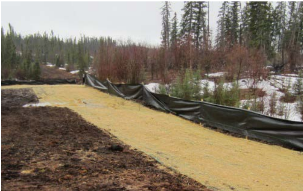
Figure 3. Sediment fence and erosion control blanket installed near the winter ice crossing at Looking Back Creek.
