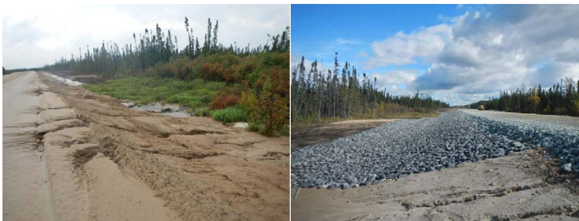
Figure 5. The unnamed tributary before and after the placement of rip rap.
