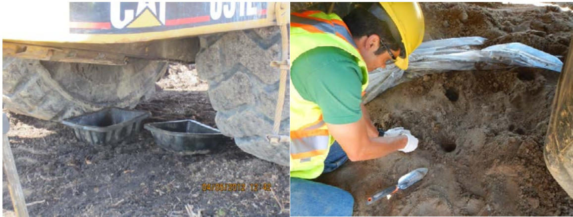
Figure 8. Mitigating potential releases using drip trays under construction equipment (left) and collecting soil samples after a hydraulic fluid release (right).
