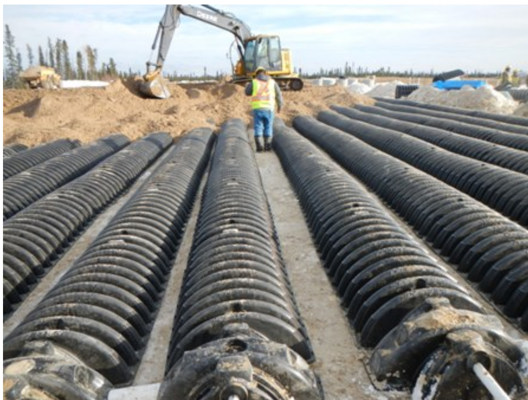
Figure 7. Filtration chambers in the drainage field being backfilled.
