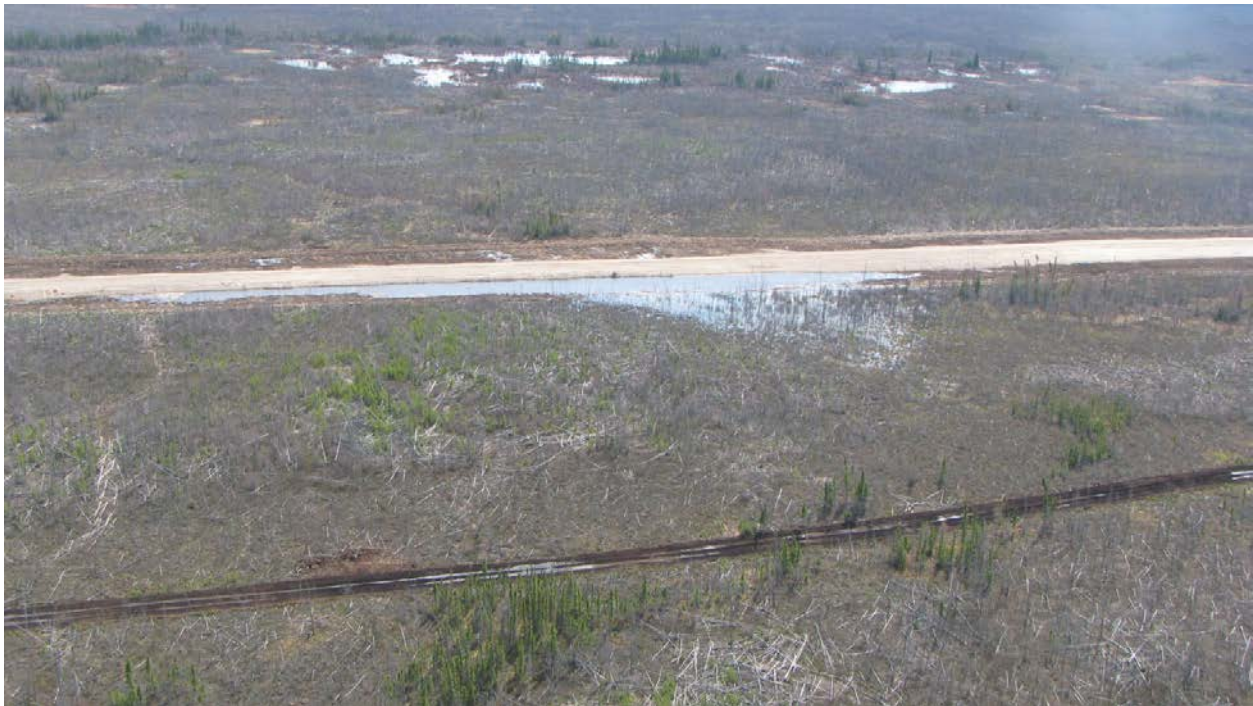
Photo 3-2: Ponding of Water Along the KIP Road ROW During Construction (May 2012).
