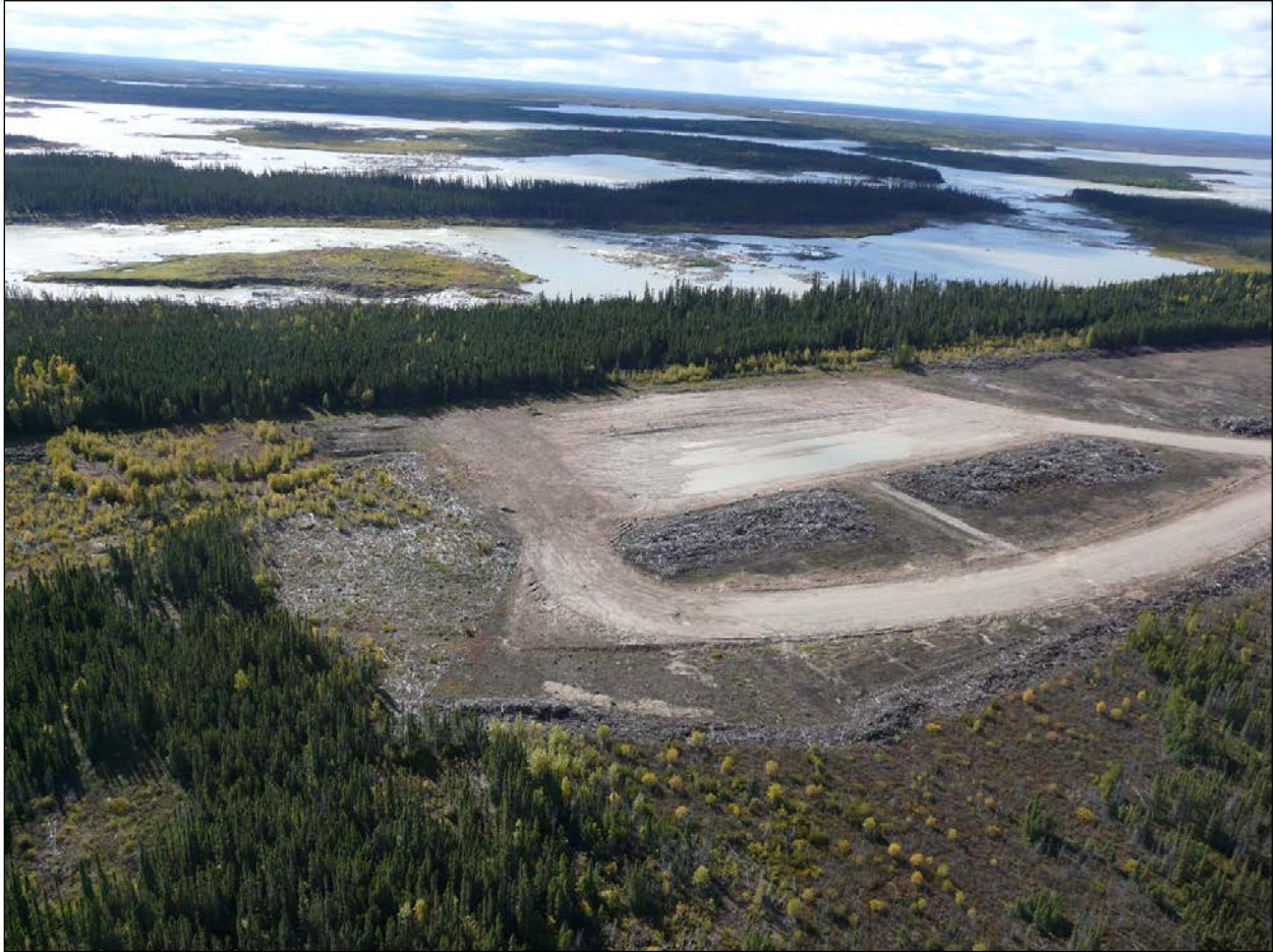
Figure 2-9: Clearing and grading at south end of Main Camp – Phase 1 (September 20, 2012).
