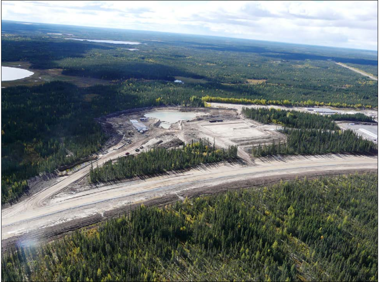
Figure 2-3: Borrow area adjacent to the start-up camp and work area (September 20, 2012).
