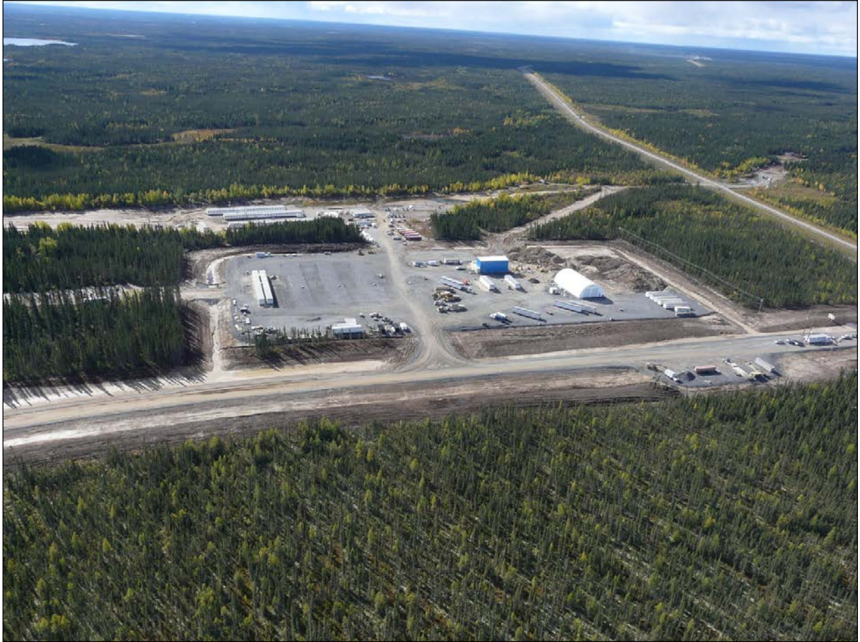
Figure 2-2: Start-up camp and work area near PR 280 (September 20, 2012).
