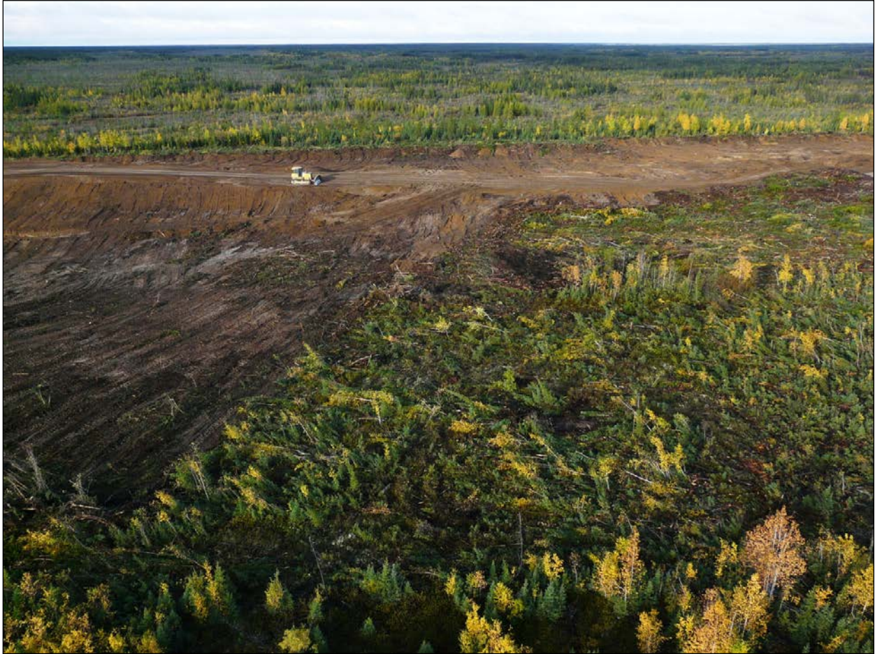
Figure 2-4: Clearing and excavation underway at G-5 borrow area (September 20, 2012).
