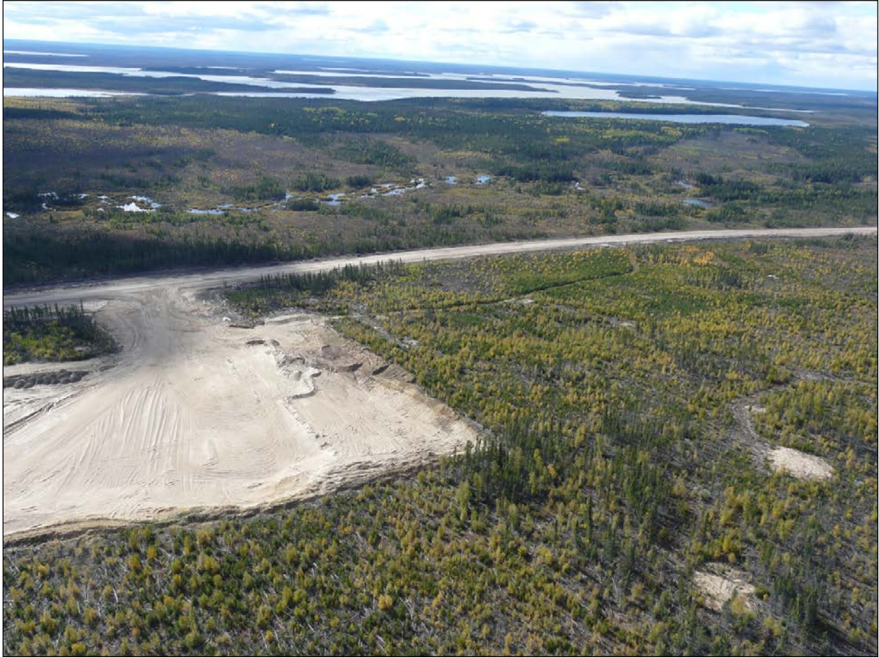
Figure 2-6: Clearing and excavation in G-1 borrow area, and nearby geotechnical test sites (September 20, 2012).
