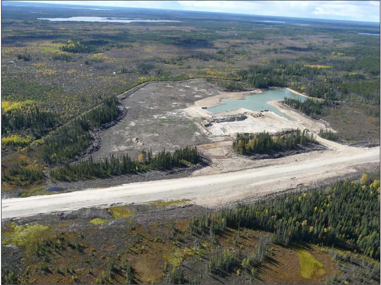
Figure 2-8: Clearing and excavation in borrow area approximately 9 km from PR 280 (September 20, 2012).
