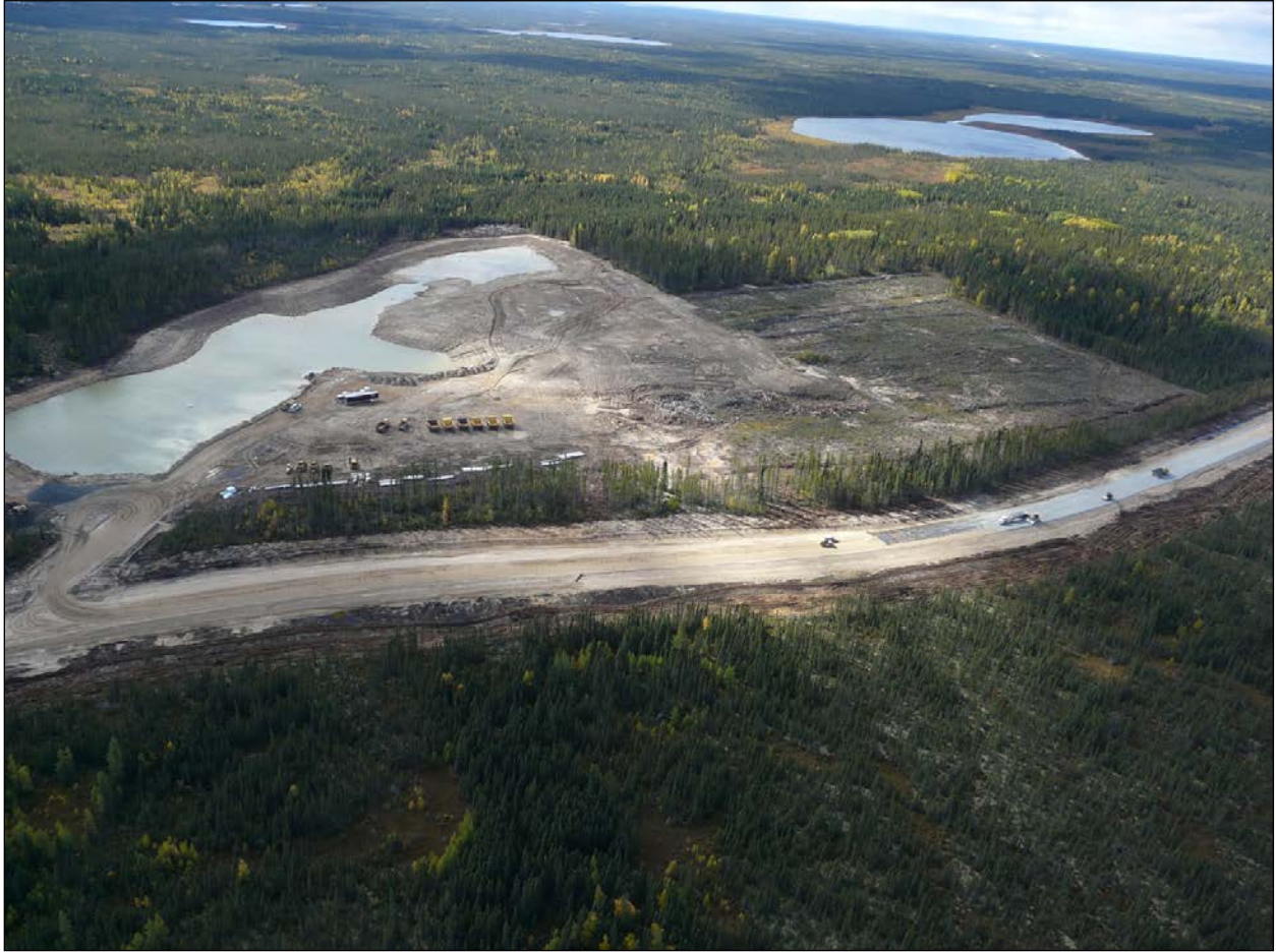
Figure 2-7: Clearing and excavation in borrow area approximately 3 km from PR 280 (September 20, 2012).
