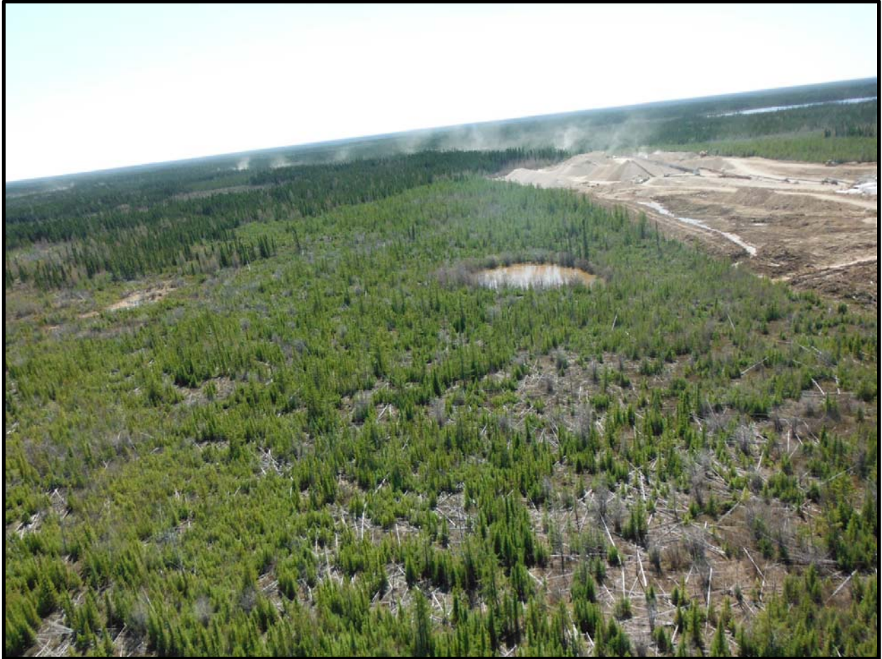
Photo D-4: Wetland (KIPS21) with Elevated Sediment Concentration in 2013, Near Active Borrow Area
