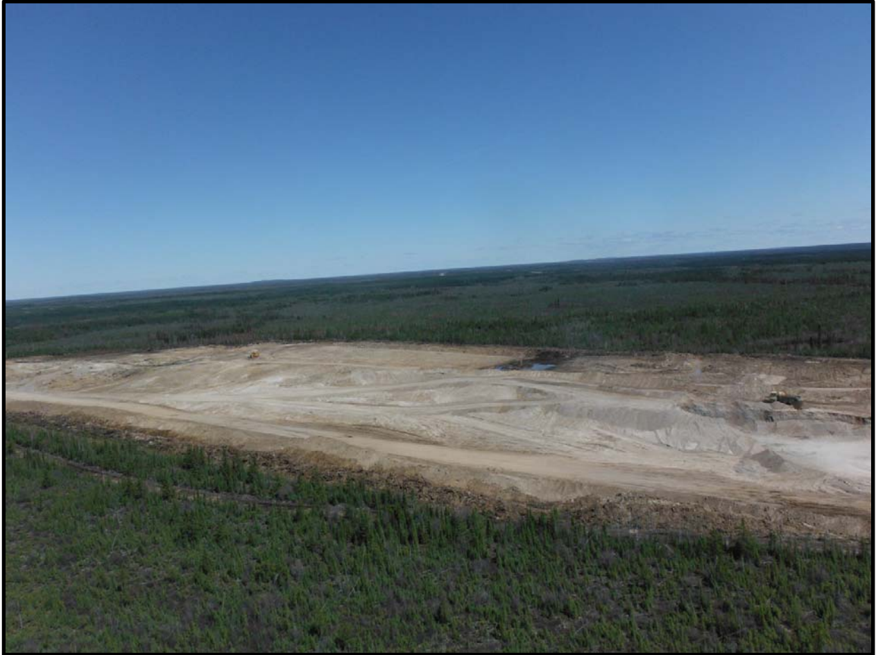
Photo D-6: Removal of Vegetation for the Development of a Borrow Area
