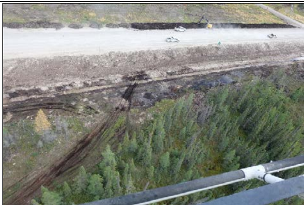
Access road ditch work
