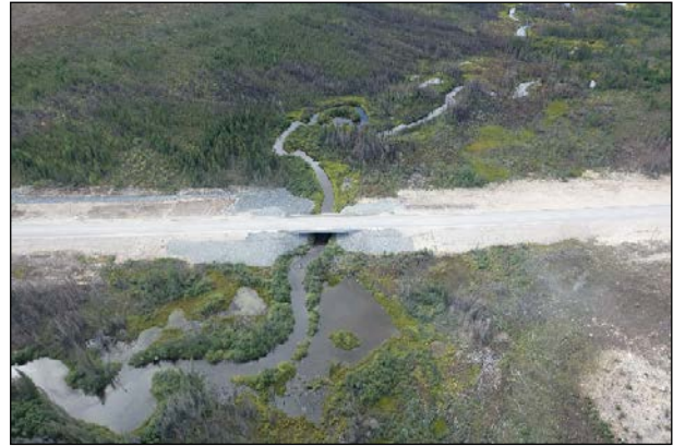
Bridge at Looking Back Creek
