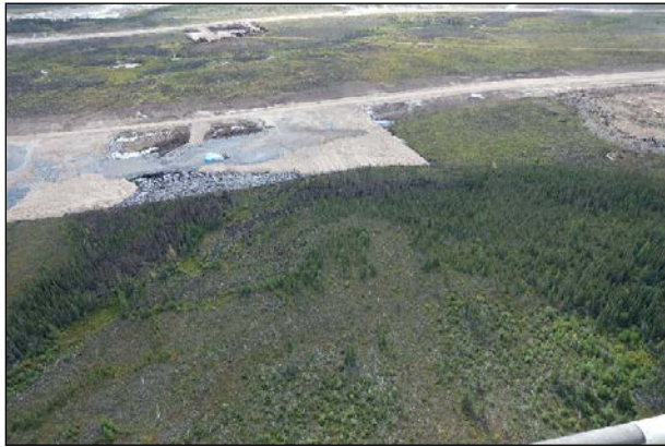
Work Area A
