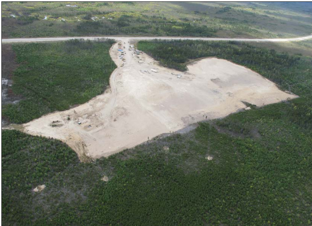
Figure 3-7: Clearing and excavation in KM-15 borrow area, west side of G-1 (September 9, 2014).
