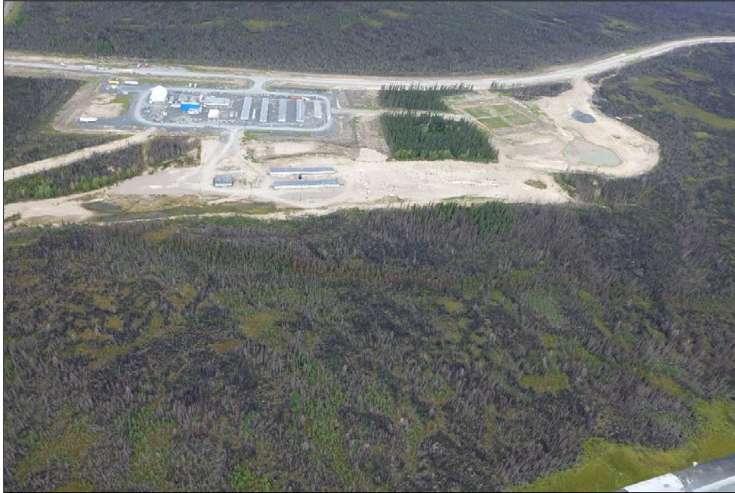
Figure 3-2: Start-up camp and work area near PR 280 (September 9, 2014).
