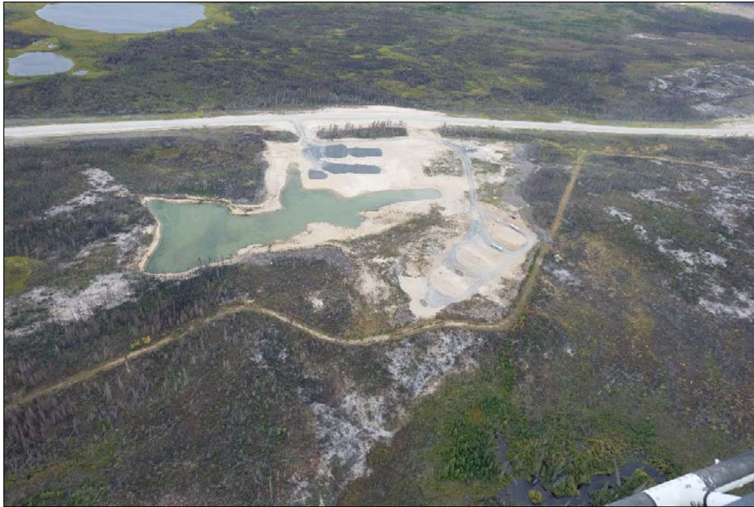
Figure 3-6: Clearing and ponding in KM-9 borrow area (September 9, 2014).
