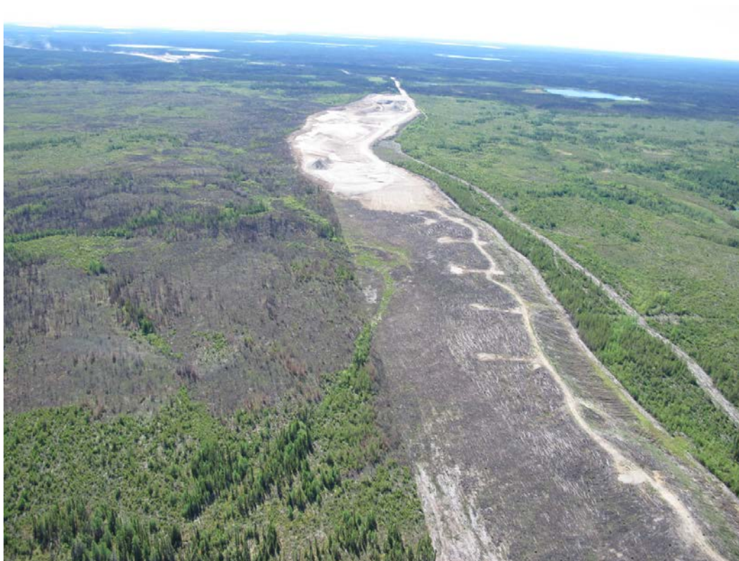
Figure 3-15: View of the borrow area G-5 north of PR280, from the north looking south, with burned forest on the east (left) side and unburned forest on the west (right) side (June 25, 2014).
