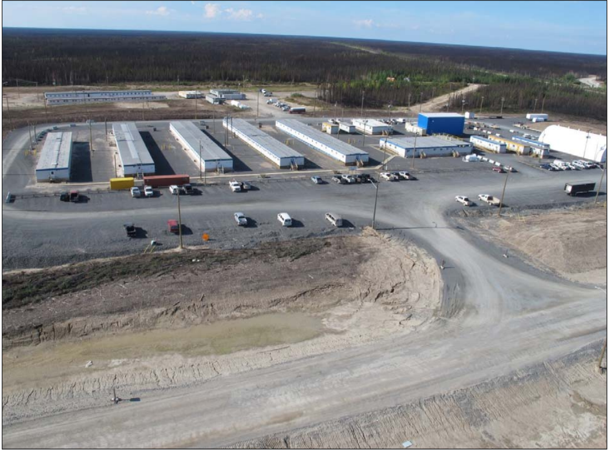
Figure 3-2: Start-up camp and work area near PR 280 (September 2, 2013).
