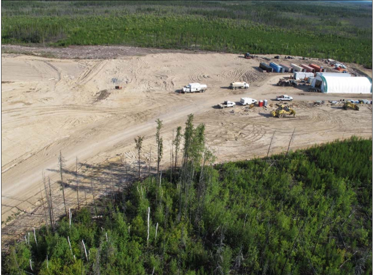
Figure 3-5: Clearing and excavation in G-1 borrow area, west side clearing (September 2, 2013).
