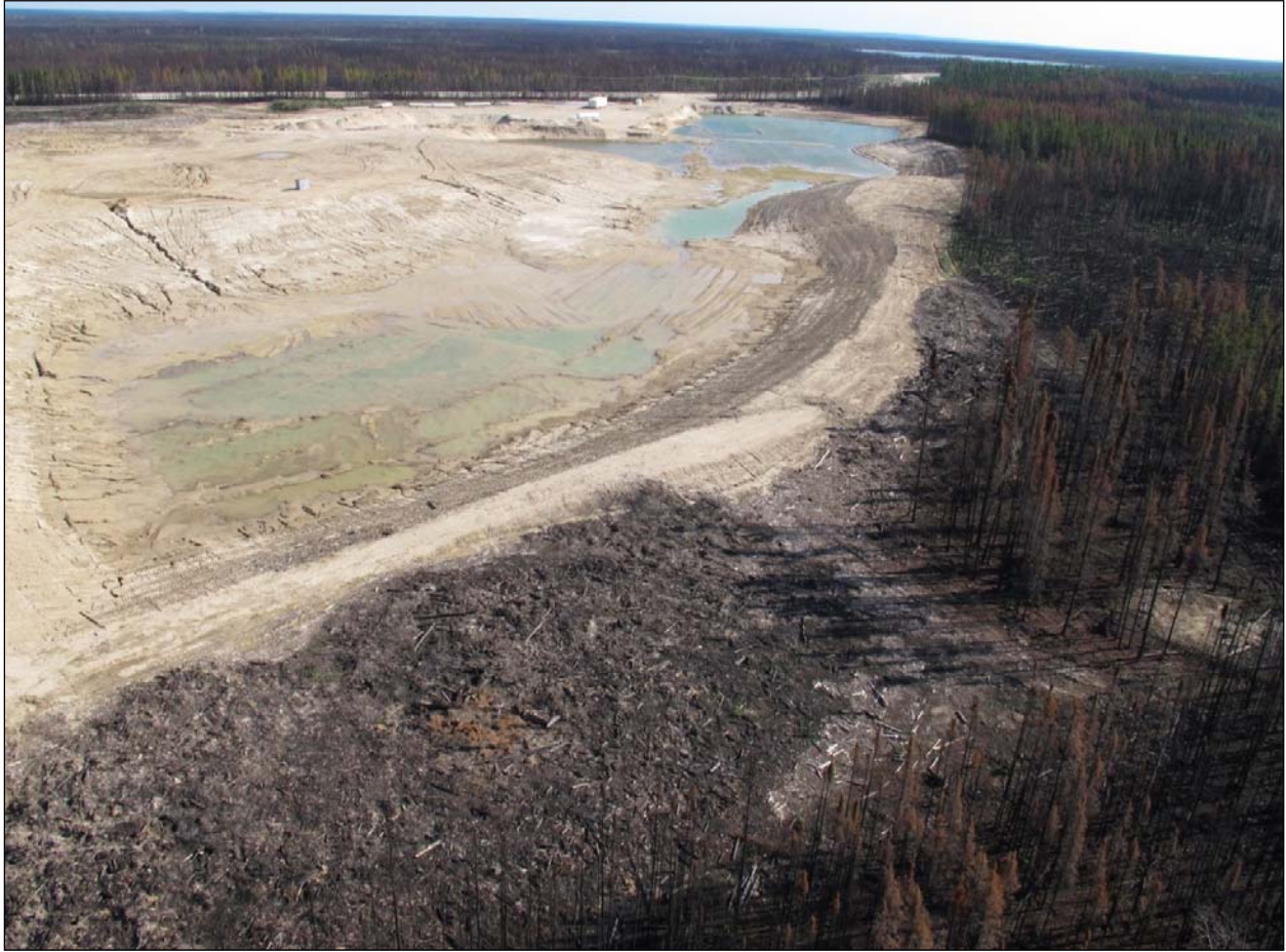
Figure 3-7: Clearing and excavation in borrow area approximately 4 km from PR 280 (September 2, 2013).
