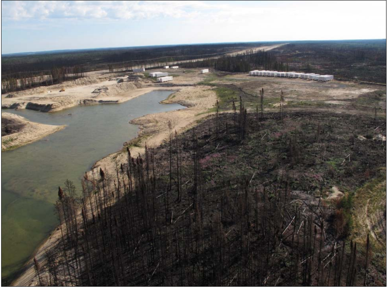
Figure 3-8: Clearing and excavation in borrow area approximately 9 km from PR 280 (September 2, 2013).
