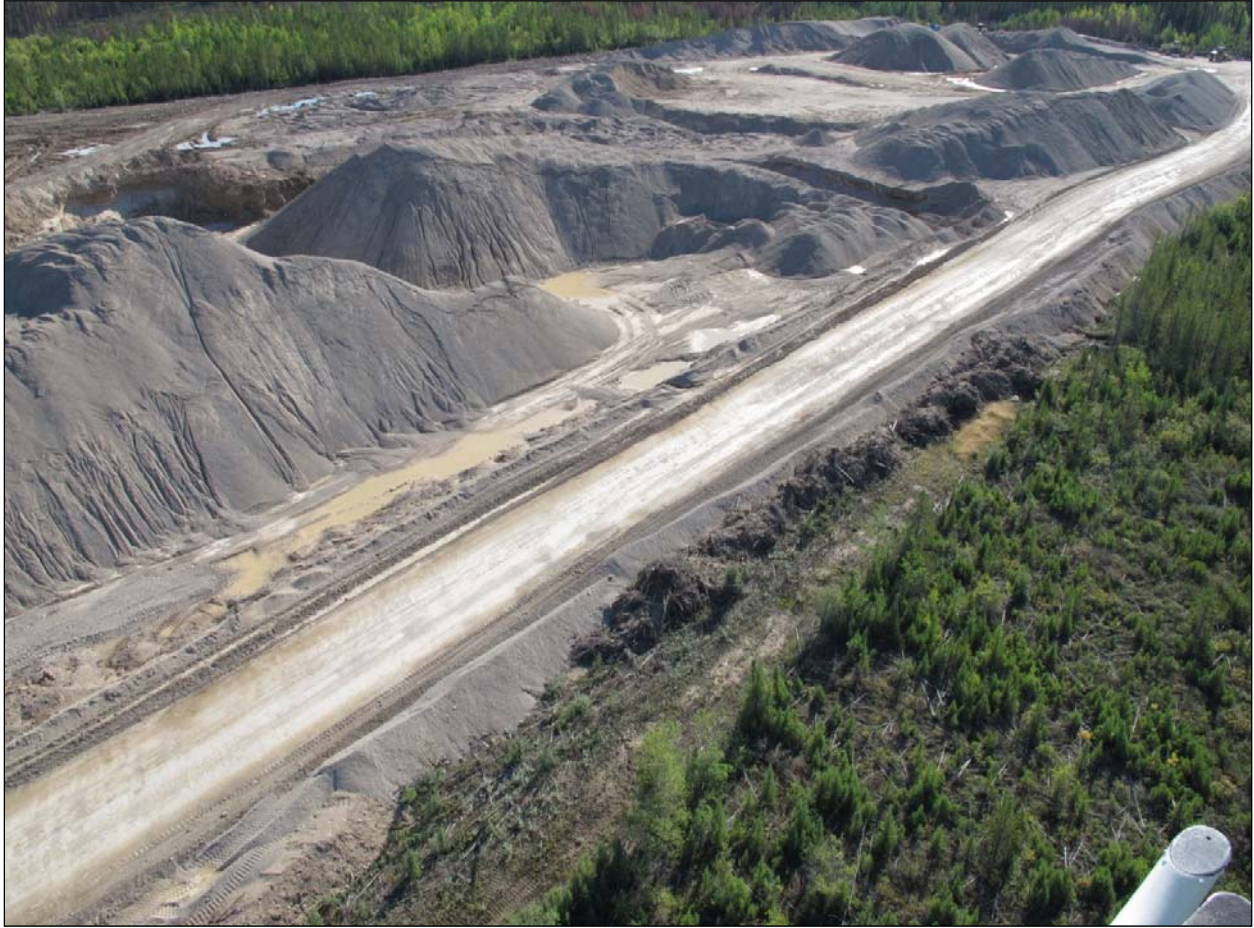
Figure 3-4: Clearing and excavation at G-5 borrow area (September 2, 2013).
