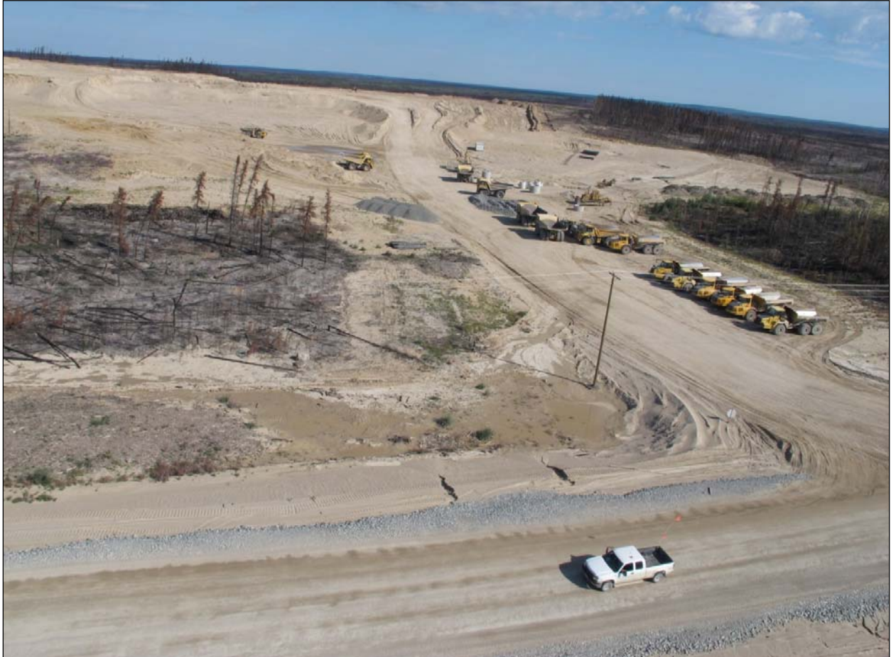
Figure 3-6: Clearing and excavation in G-1 borrow area, east side clearing (September 2, 2013).
