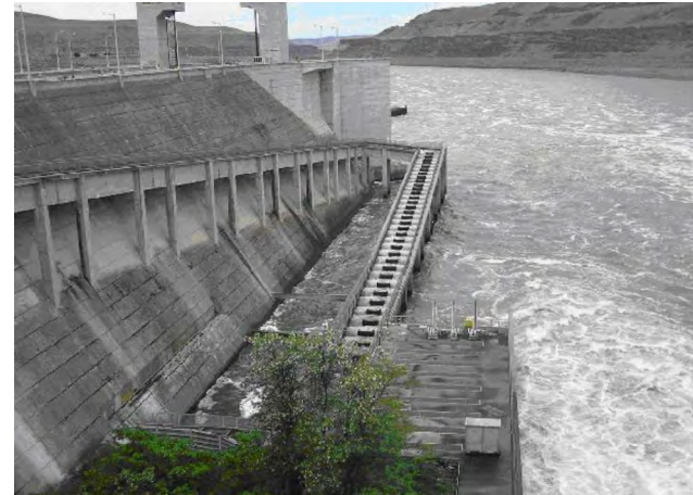
PHOTO 4 LOWER MONUMENTAL SOUTH LADDER SHOWING FISHWAY ASCENDING DAM
