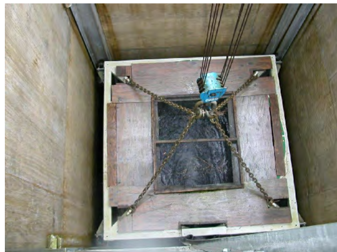
HOPPER STYLE FISH LIFT
