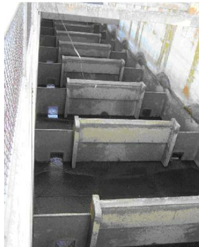
PHOTO 1 THE DALLES DAM, EAST BANK ICE HARBOR STYLE FISHLADDER, SHOWN DEWATERED
