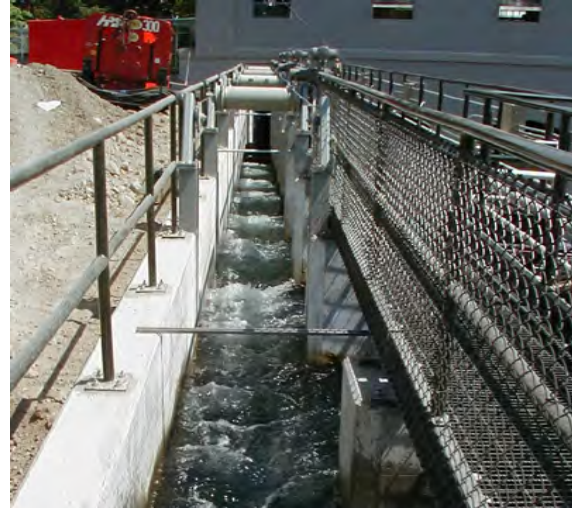
PHOTO 3 RIVER MILL DAM FISHWAY EXIT SECTION (TO RESERVOIR) SHOWING ADJUSTABLE CONTROL WEIRS TO ACCOMMODATE VARYING POOL ELEVATION
