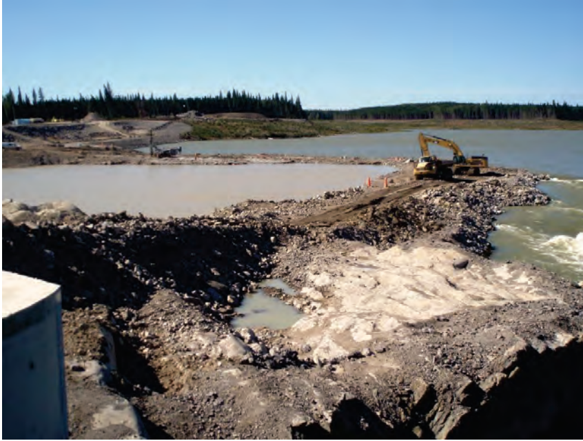
Photograph 3-7: Cofferdam Removal 'in the wet' (Wuskwatim Project, Manitoba Hydro, 2011)
