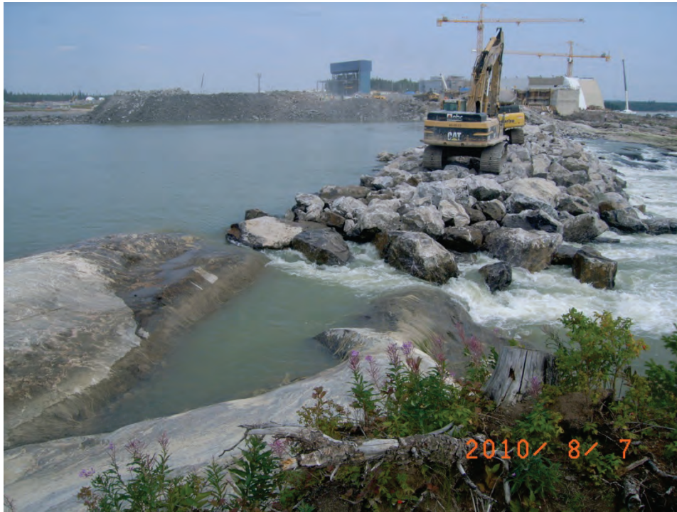
Photograph 3-6: Progressive Rock Fill Cofferdam (Wuskwatim Project, Manitoba Hydro, 2010)
