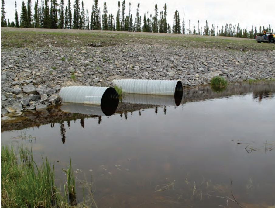
Photograph 2-1: Typical access road stream crossing (Wuskwatim Access Road, Manitoba Hydro, 2011)
