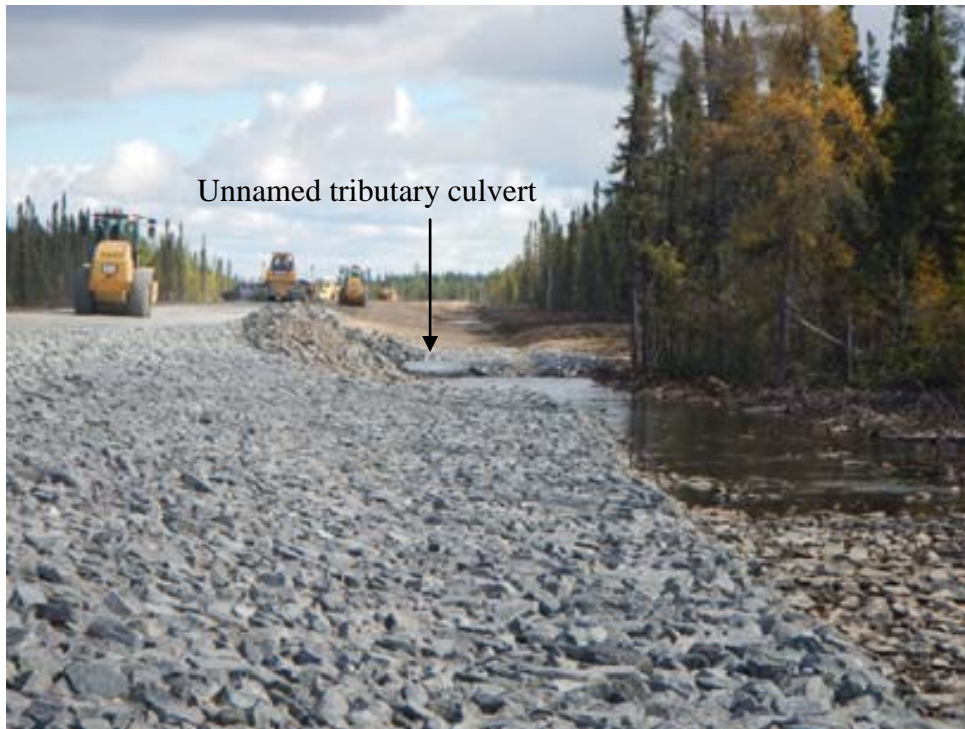
Figure 5. Erosion control (rip rap) complete along ditches and banks of the unnamed tributary.
