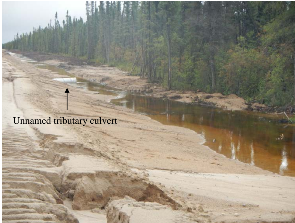
Figure 3. Area in vicinity of the culvert crossing during construction.
