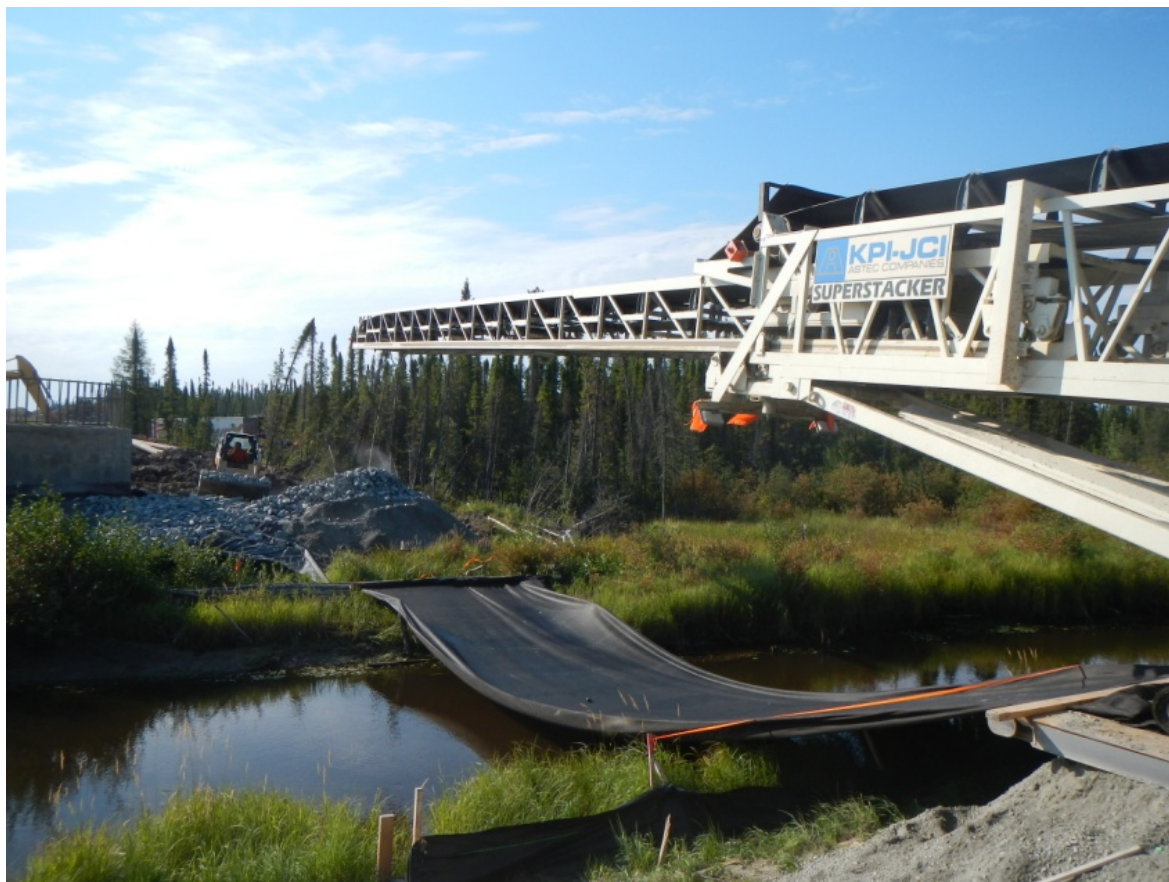
Figure 2. Conveyor belt moving material from the north to south side of Looking Back Creek at the crossing location.
