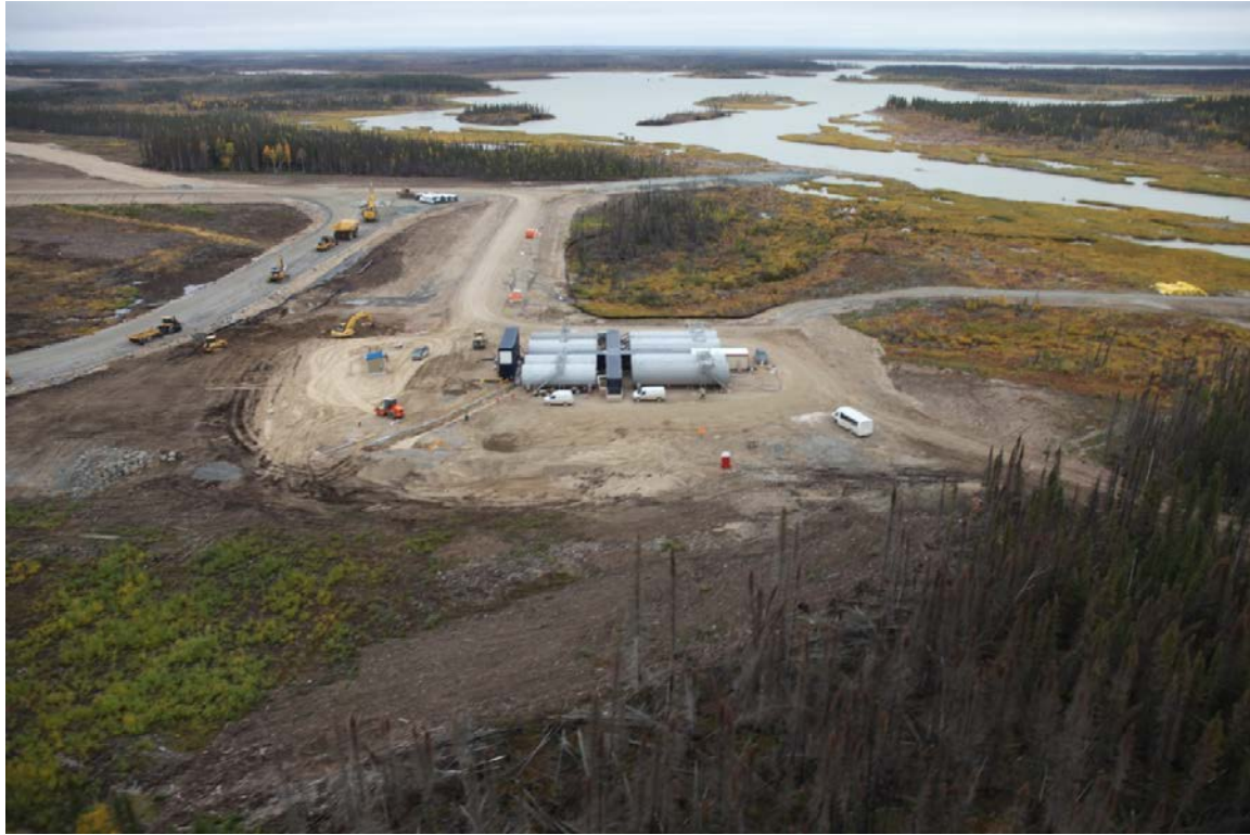
Figure 2: Aerial photo of the Wastewater Treatment Plant
