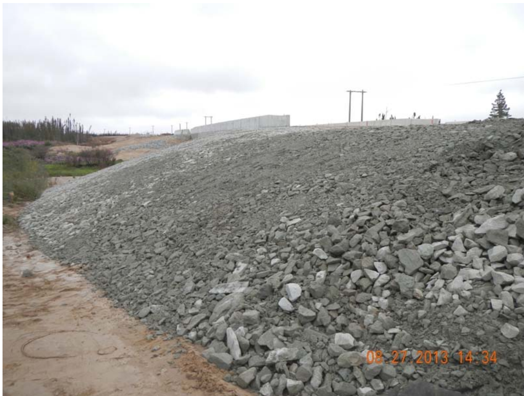
Figure 5: Rip rap on the embankment approaching Looking Back Creek.
