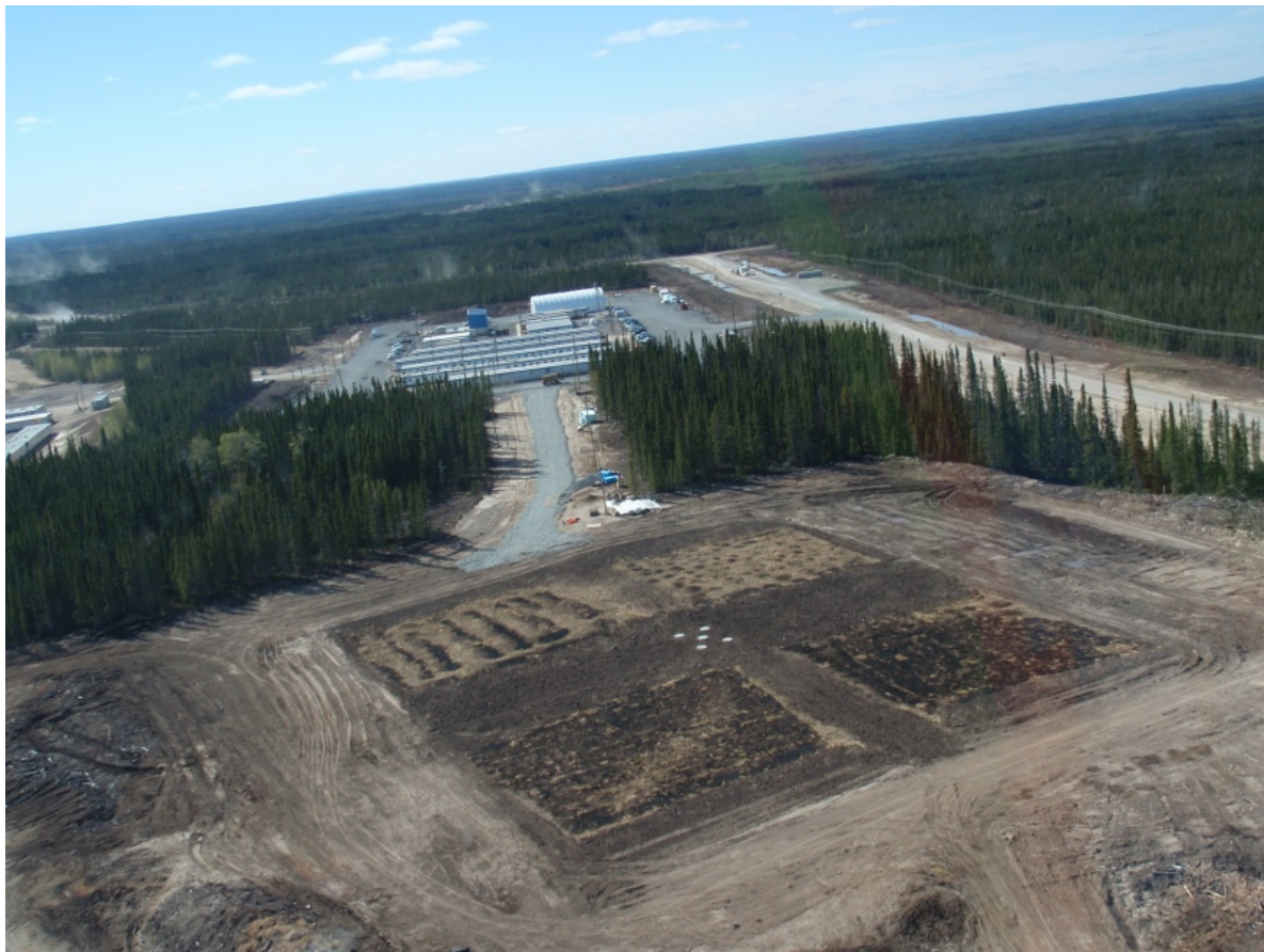
Figure 6: Start-up camp wastewater drain field.
