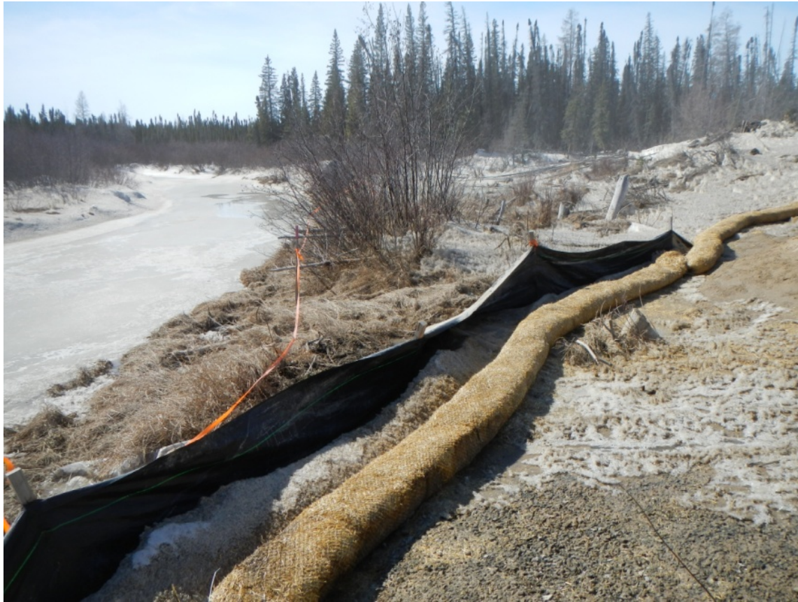
Figure 3: Straw rolls installed at Looking Back Creek.
