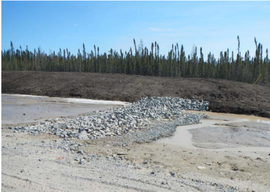
Figure 4: A ditch check along the access road.
