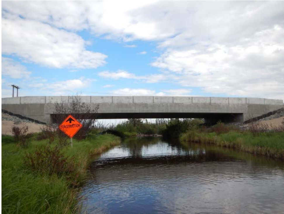
Figure 1: Clear-span bridge over Looking Back Creek.
