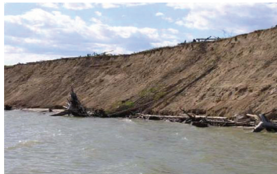
PHOTO 3-12 Shoreline erosion along the banks of the Limestone Forebay.
