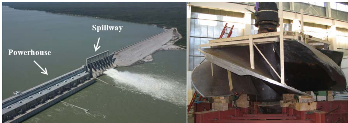
Generating station showing the powerhouse and spillway Water passing through the powerhouse turns turbines (example turbine on right).
