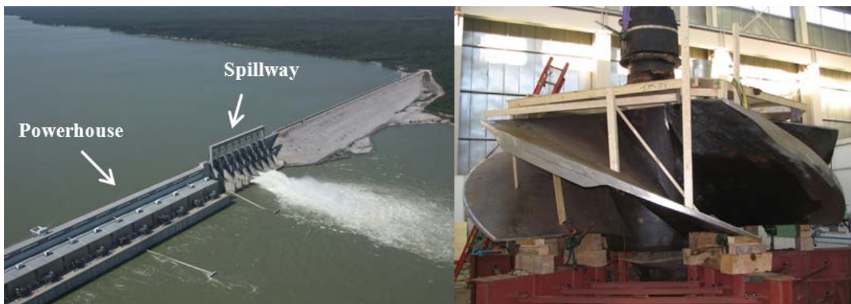
Generating station showing powerhouse and spillway. Water passing through the powerhouse turns turbines (example turbine on right).
