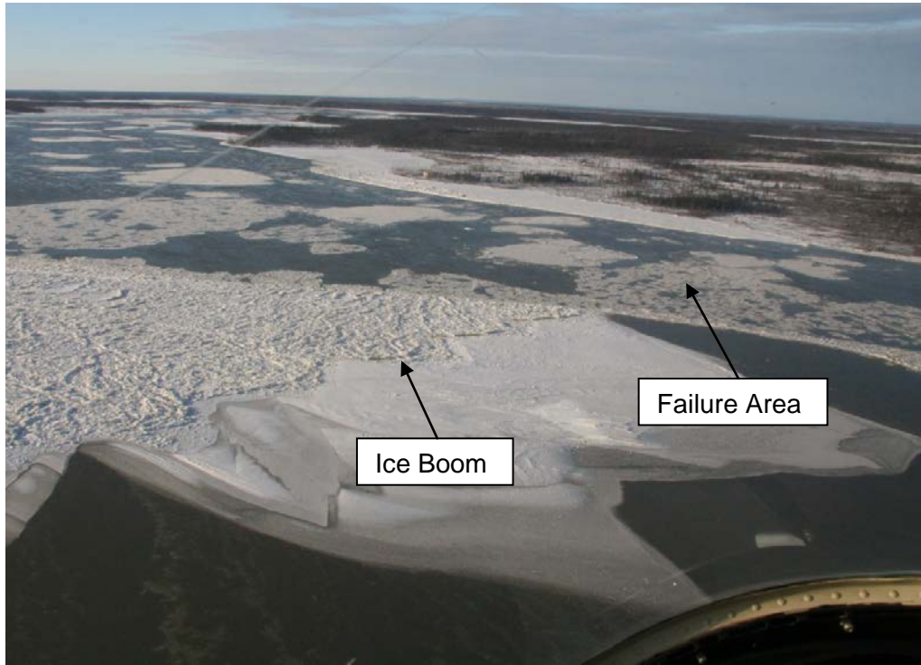
Photo 5: Ice Flowing Past the Failed Ice Boom
