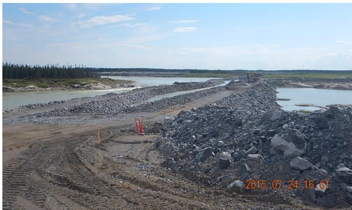
Figure 3: Central Dam Cofferdam outer rock groin in progress
