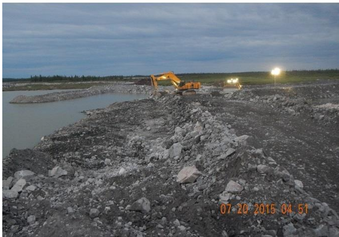
Figure 2: Central Dam Cofferdam outer rock groin construction
