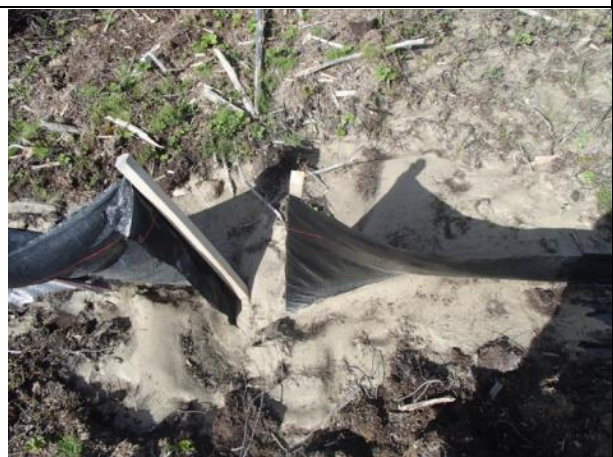
Siltation leak through fence
