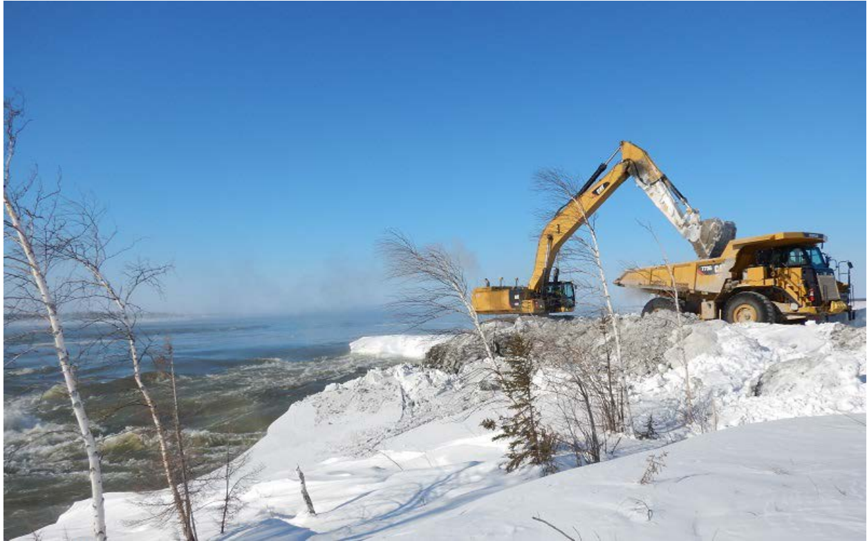
Figure 20: Excavator placing material removed from the North Channel Rock Groin Extension into a haul truck on March 11, 2017
