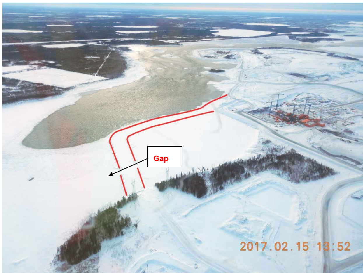
Figure 13: Aerial view of the Tailrace Summer Level Cofferdam in the winter, showing the inner and outer rock groins (red lines) and gap left for fish movement.
