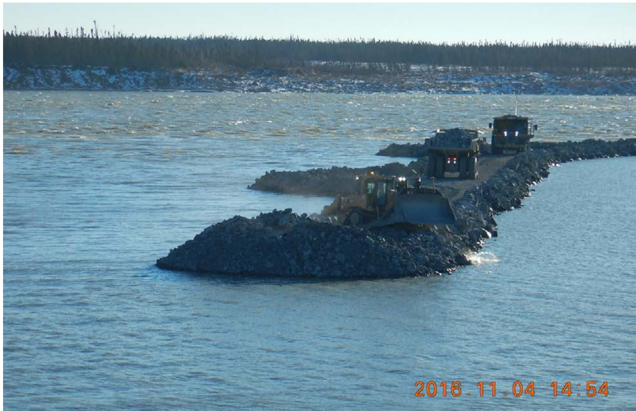
Figure 11: Placement of Class C1/C2 rockfill and riprap on the outer groin of the Tailrace Summer Level Cofferdam on November 4, 2016
