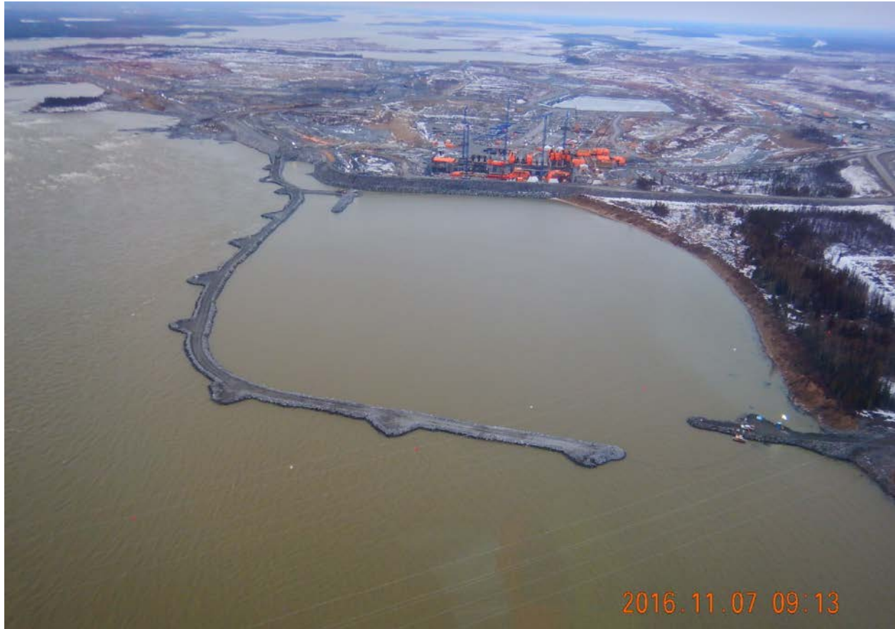
Figure 12: Aerial view of the incomplete Tailrace Summer Level Cofferdam, showing the outer rock groin (extending from the left) and a spur of the inner rock groin (extending from the right) on November 7, 2016
