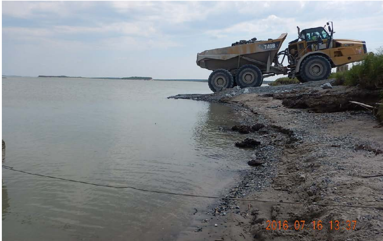
Figure 7: Cat 740 haul truck placing rock for the repair of the Downstream Boat Launch on July 16, 2016
