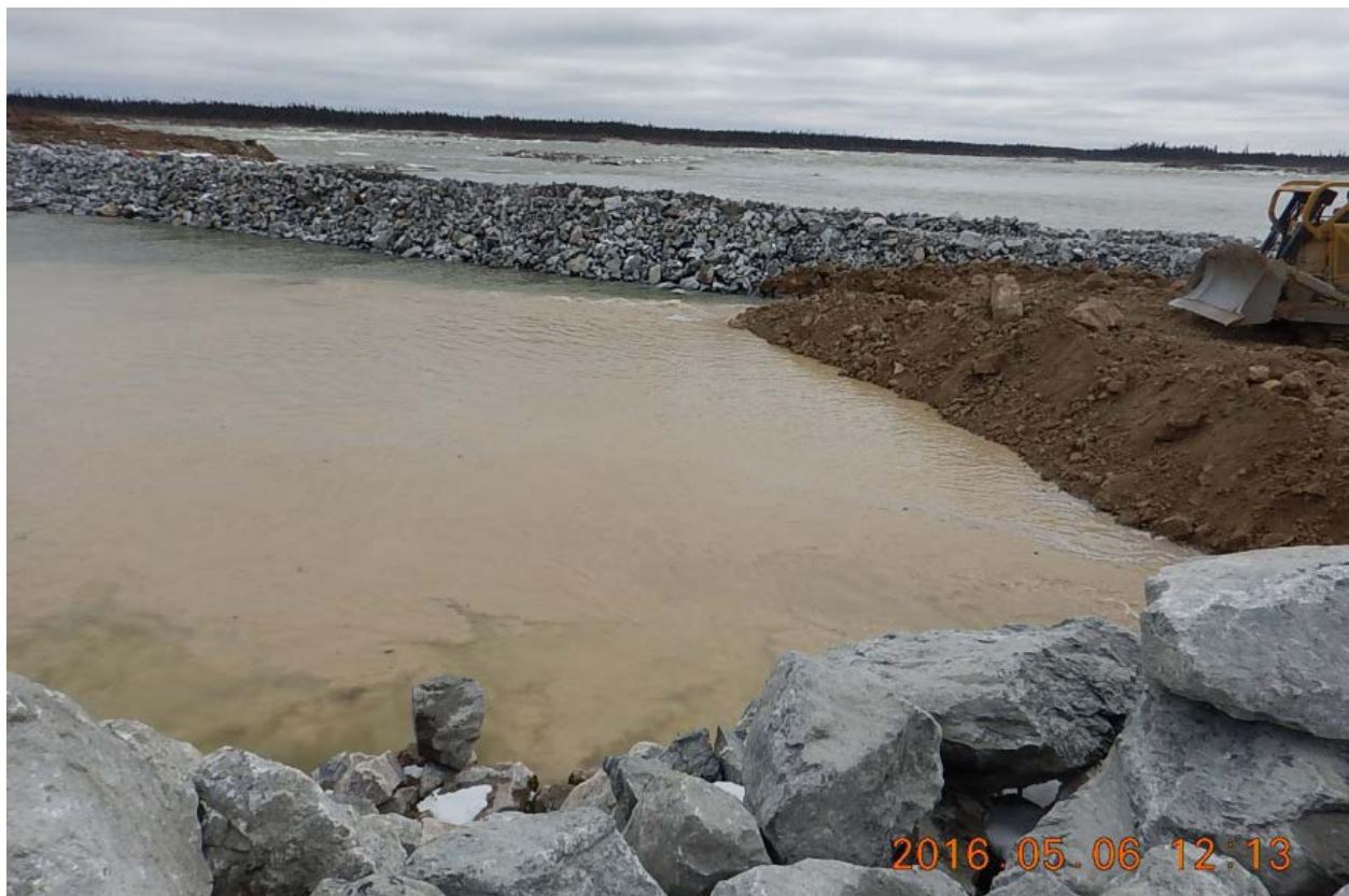
Figure 5: On May 6, 2016, a sediment plume developed while placing impervious material at the Central Dam Cofferdam Extension, which is shown in the background.
