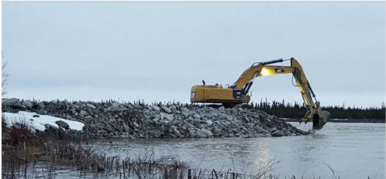
Figure 18: Excavator placing C3 material at the North Channel Rock Groin Extension on November 14, 2016
