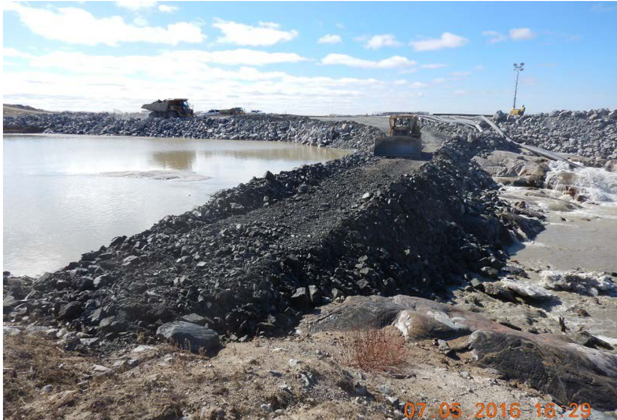
Figure 6: Dozer placing coarse rockfill to create a barrier to prevent impervious material from entering the river (May 7, 2016)
