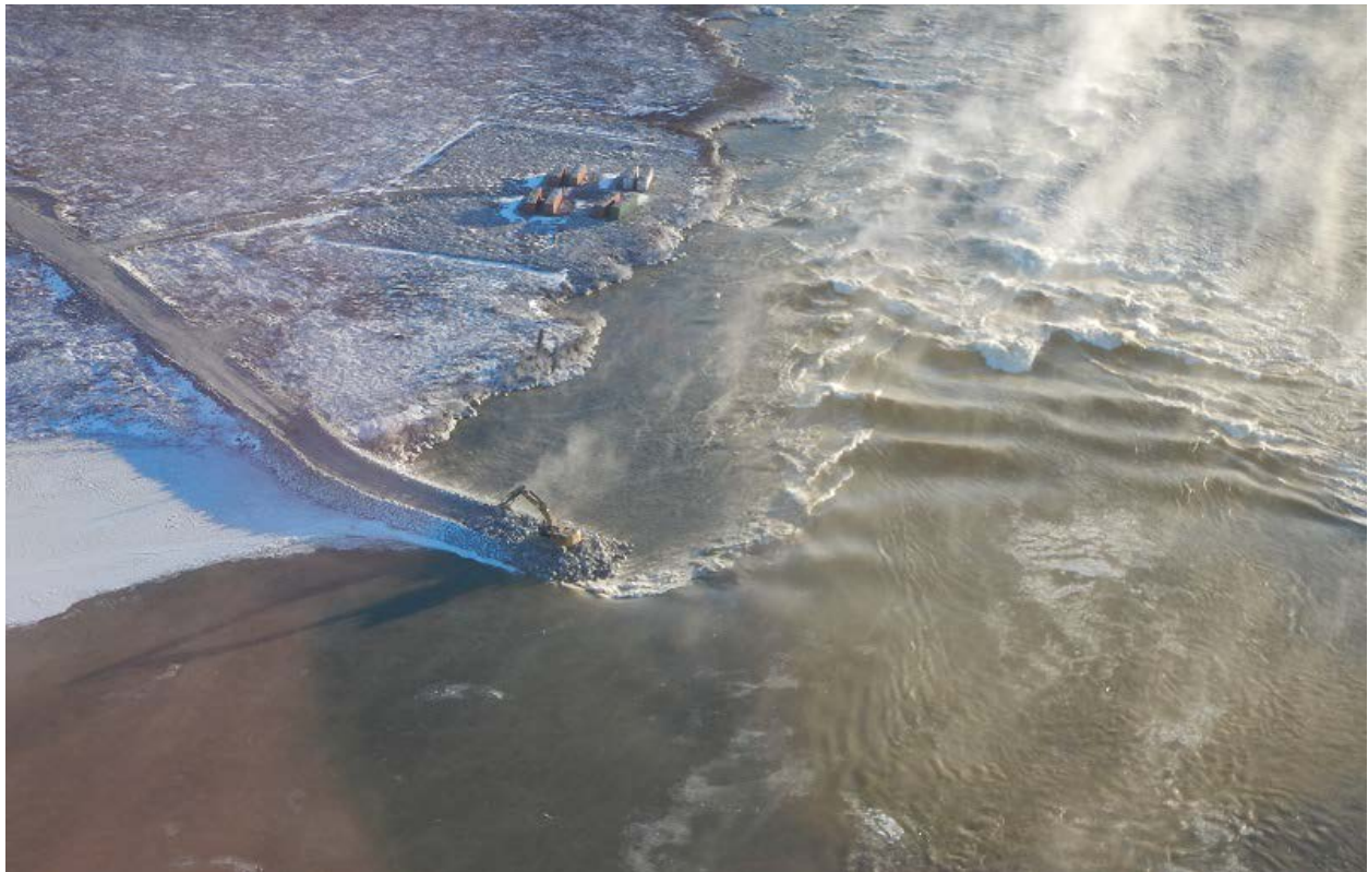
Figure 19: Aerial view of a Cat 390D excavator placing C3 material at the North Channel Rock Groin Extension on November 19, 2016
