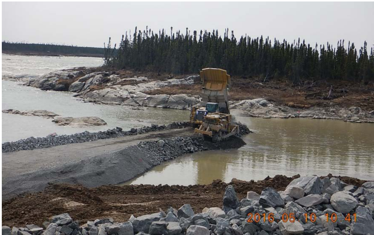
Figure 4: Constructing a rock groin for the Central Dam Cofferdam Extension on May 10, 2016.
