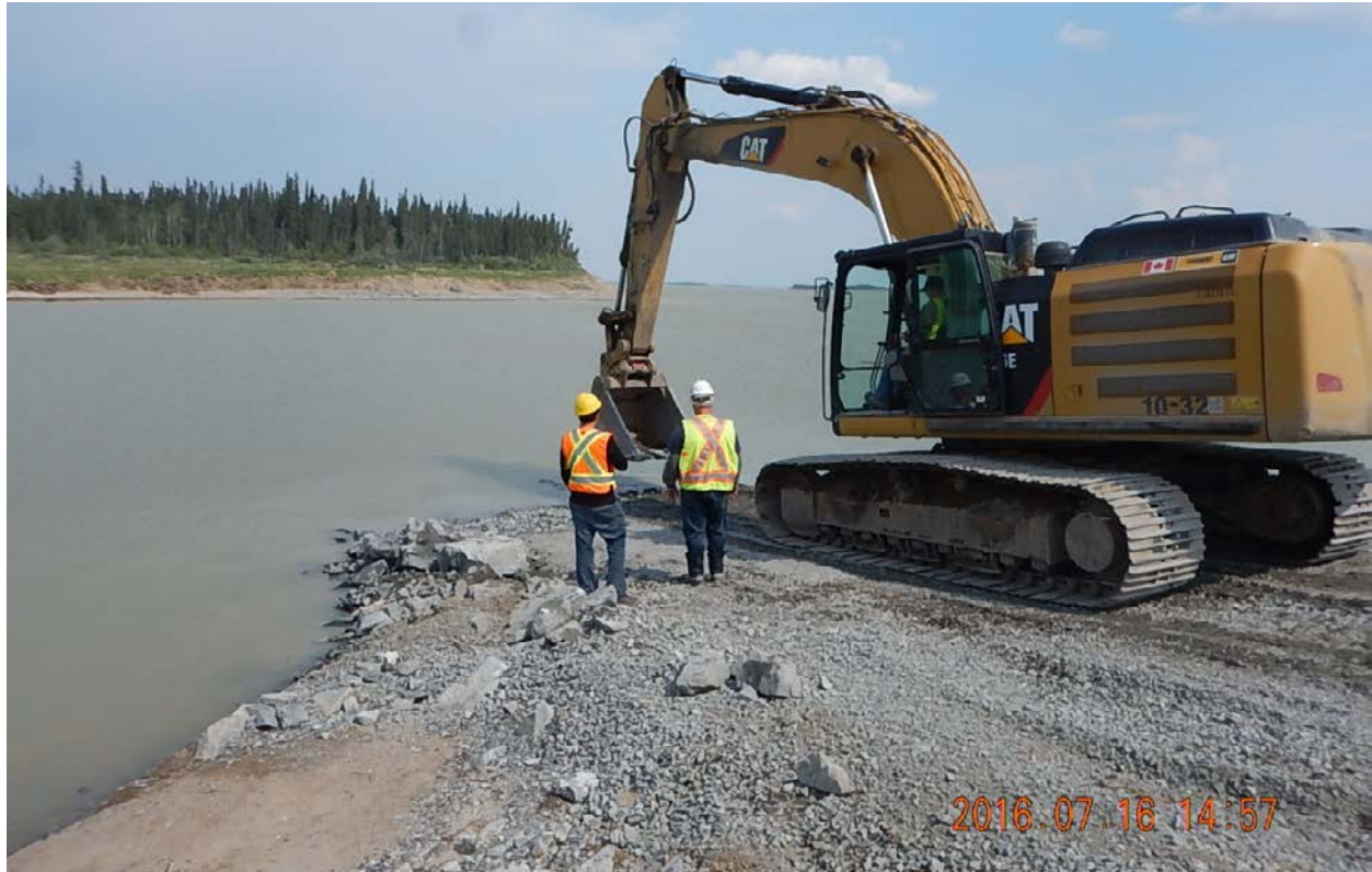
Figure 8: Excavator placing and shaping rockfill during the repair of the Downstream Boat Launch ramp on July 16, 2016
