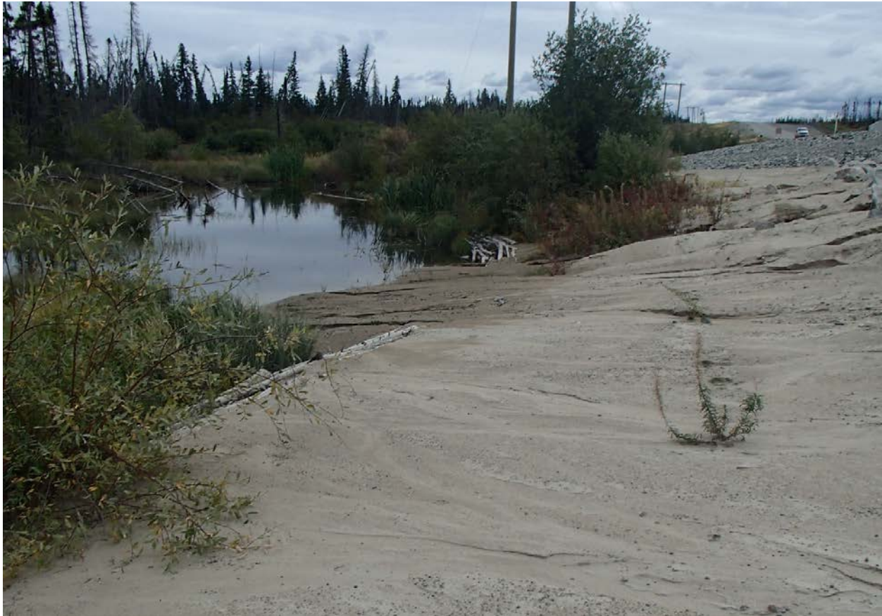
Photo 3-4: Erosion and sedimentation from North Access Road into a natural waterbody adjacent to Looking Back Creek
