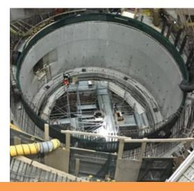
Installation of the unit 1 draft tube liner in February. This is the first of seven draft tube liners that will be installed. Draft tube liners are giant steel pipes that separate the concrete structure from the water that flows through them – the liners help prevent erosion to the concrete.
