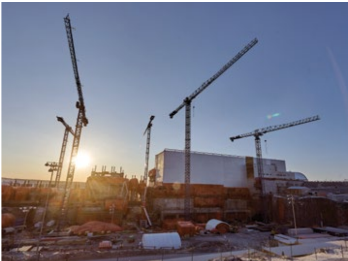
Concrete work was accomplished over the coldest winter months on the exterior portion of the Keeyask Powerhouse complex with the use of hording (orange tarps). Units 1, 2 and 3 and the Service Bay are now enclosed.
