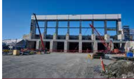
Mar. 23, 2018 Gate installation
