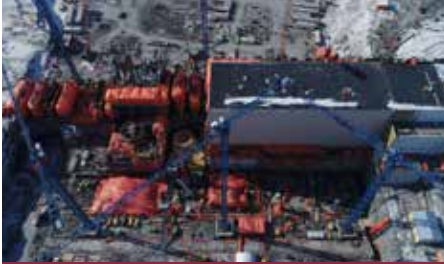
Jan. 26, 2018 Units 2 and 3 Enclosure
