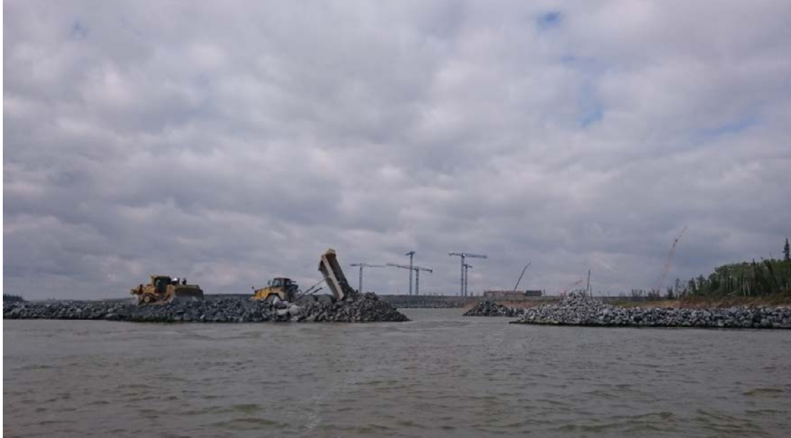
Figure 9: A Komatsu HM400 haul truck delivering rockfill to close the outer groin of the Tailrace Cofferdam on August 20, 2017.
