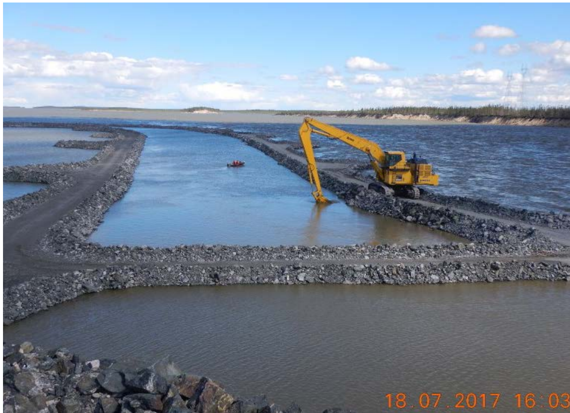
Figure 8: A Komatsu PC2000 excavator being used to carry out bedrock scraping tests to determine the extent of dredging required to remove sediment and rocks from between the groins of the Tailrace Cofferdam. Photo taken July 18, 2017
