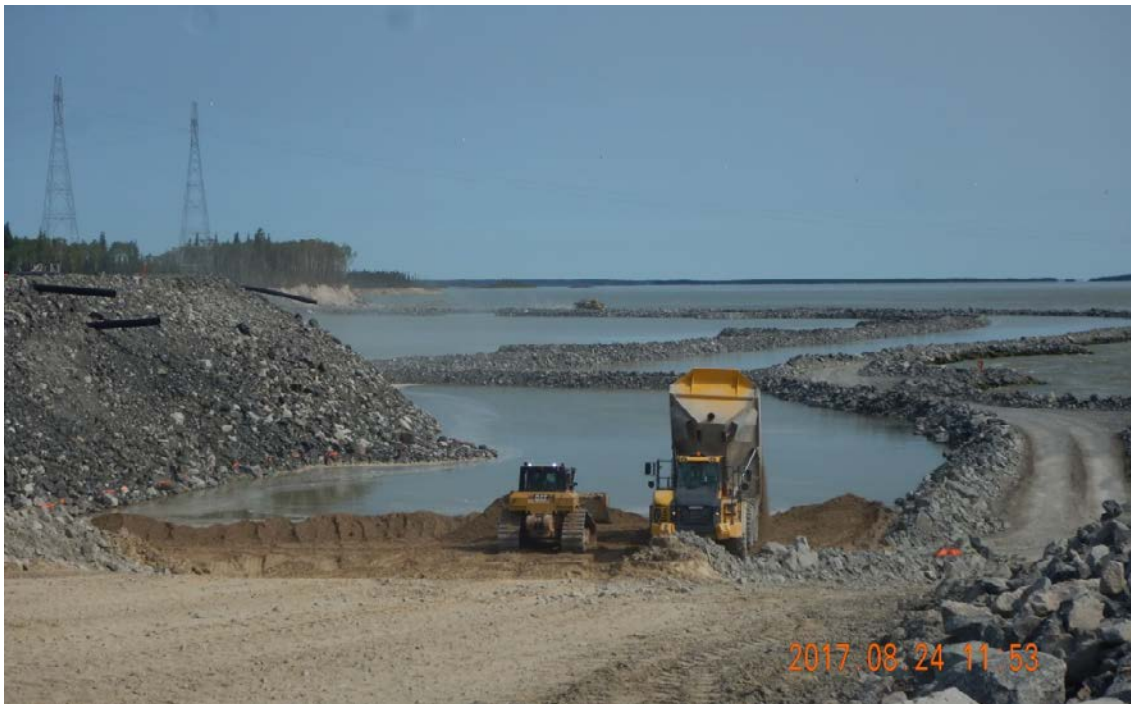
Figure 10: A Komatsu HM400 haul truck delivering sandy-silt material for placement by a Cat D6T dozer to build the impervious core of the Tailrace Cofferdam on August 24, 2017
