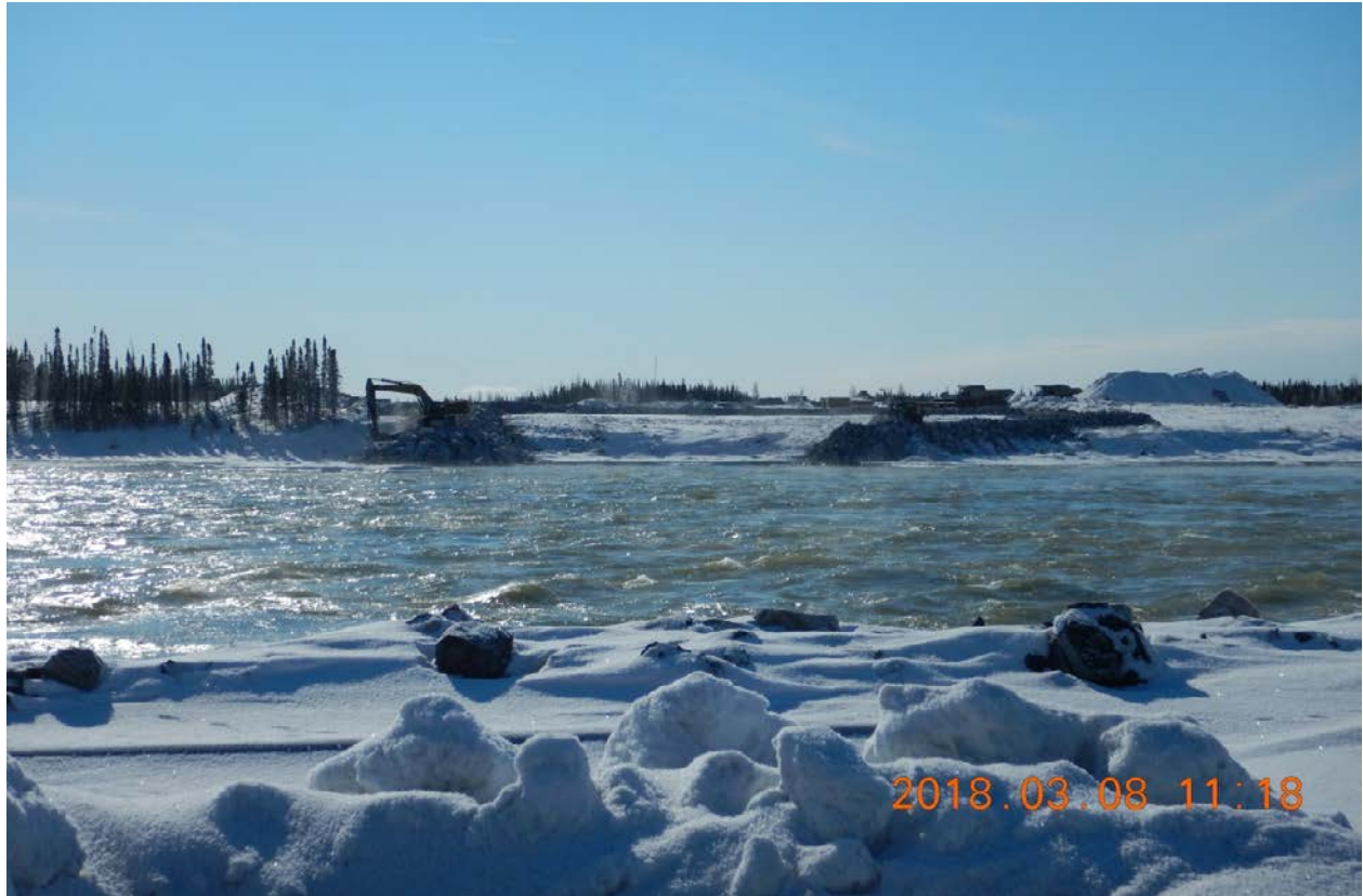
Figure 16: Construction of the Upstream and Downstream South Dam Cofferdams. A dozer places rockfill material on the upstream portion (right), while an excavator breaks ice along the shoreline and moves rockfill material into place on the downstream portion (left)
