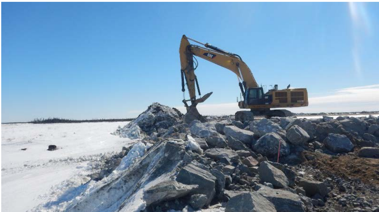
Figure 4: A Cat 390D excavator placing Class C4 rock material at the North Channel Rock Groin on April 12, 2017
