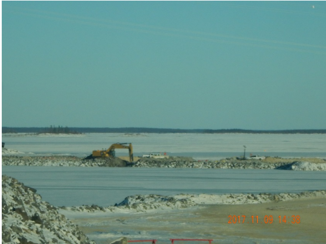
Figure 15: Photo shows an excavator removing rockfill material to create the channel
