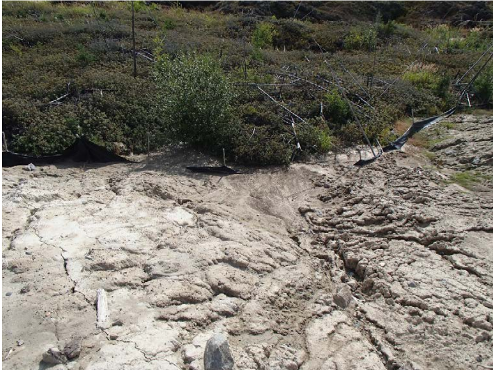
Failed silt fence on east side of EMPA D16 (looking east) on August 25, 2017
