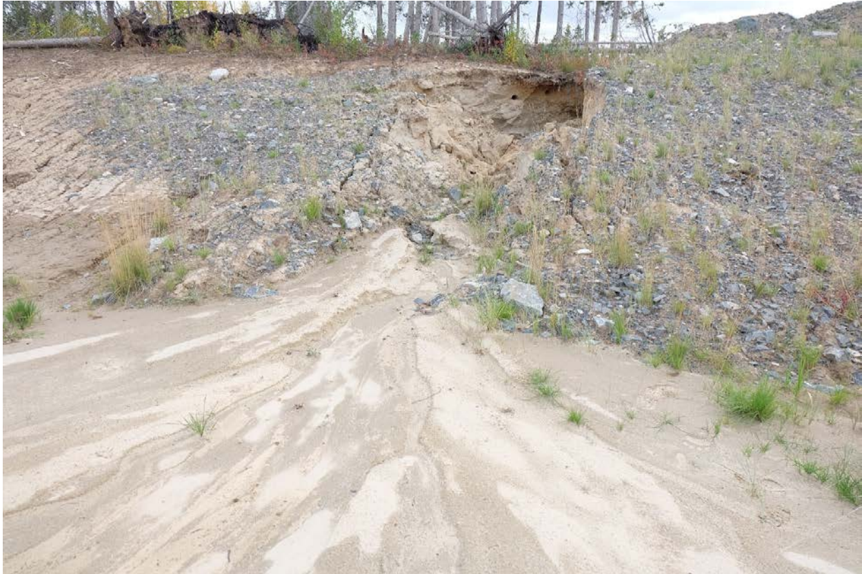
Figure 3–17: Erosion gully in NAR ditch along treed bank, September 2017
