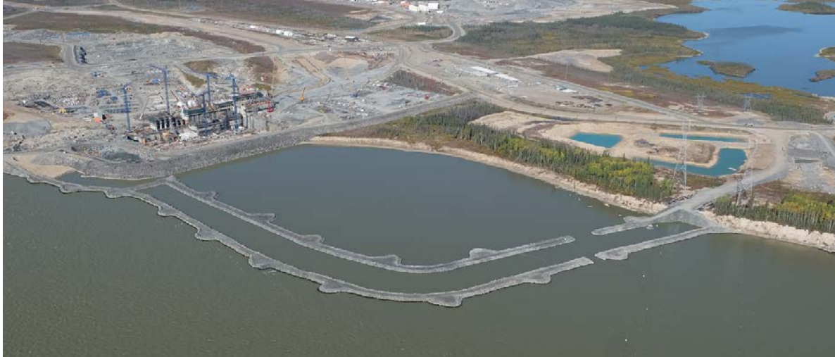
Powerhouse and tailrace channel summer cofferdam construction (looking northwest) on September 19, 2017
