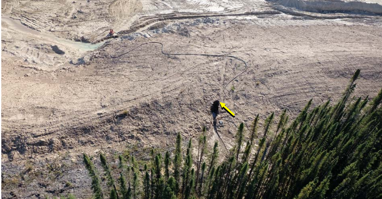
Borrow Area N-5 (looking south) on September 19, 2017. Yellow arrow identifies drainage hose and gully at location A
