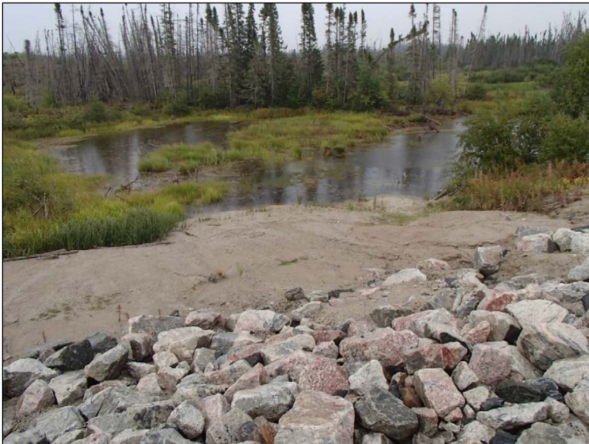
Photo 3-3: Erosion and sedimentation from the North Access Road into a natural waterbody adjacent to Looking Back Creek
