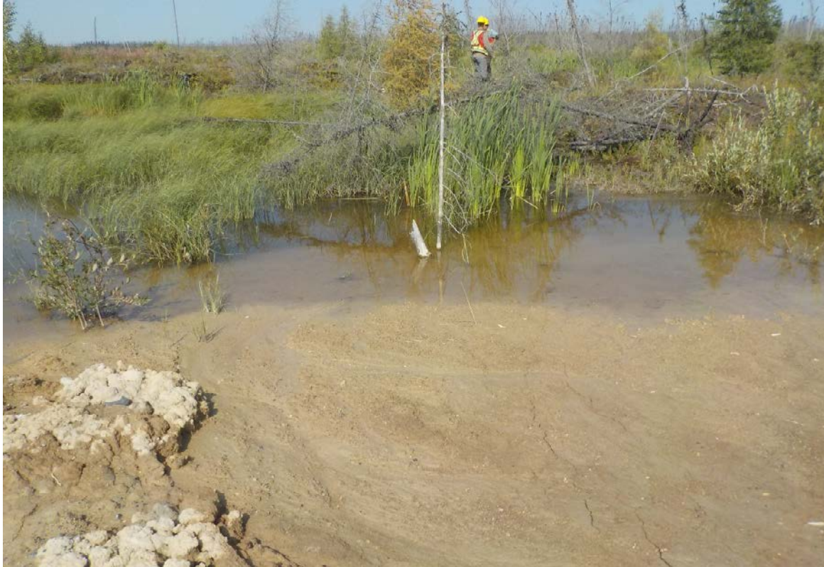
Sediment from EMPA entering the buffer of Wetland 51
