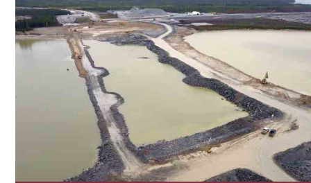
Sept. 2018 South Dam Cofferdam
