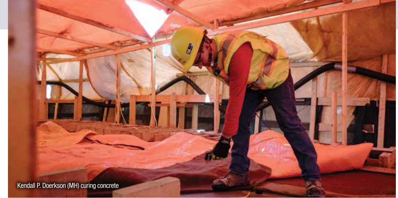
The Powerhouse enclosed with a temporary winter structure (hoarding) for winter work
