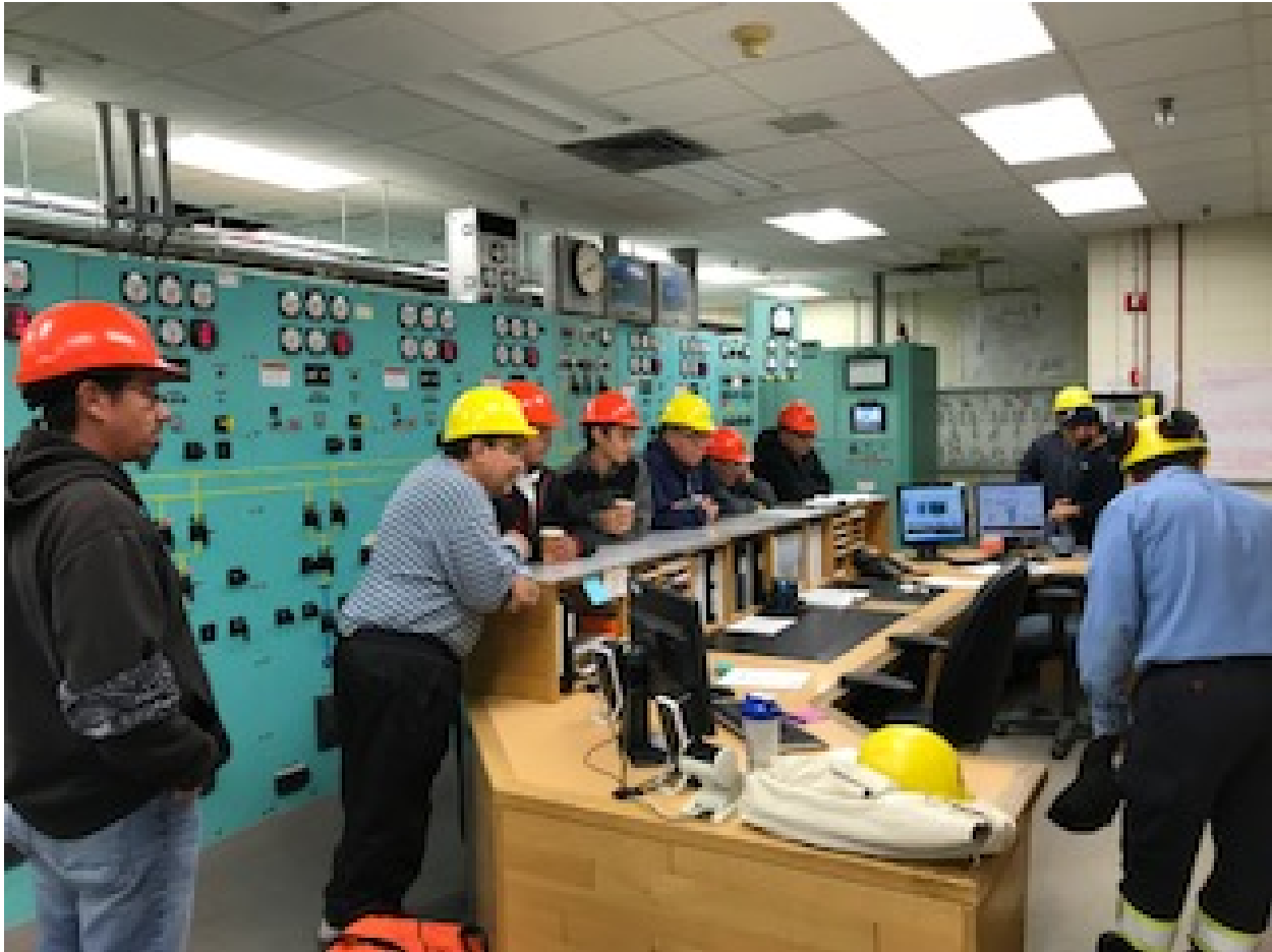
Photo 1: Inside the Kelsey Generating Station on the YFFN Waterways Tour
