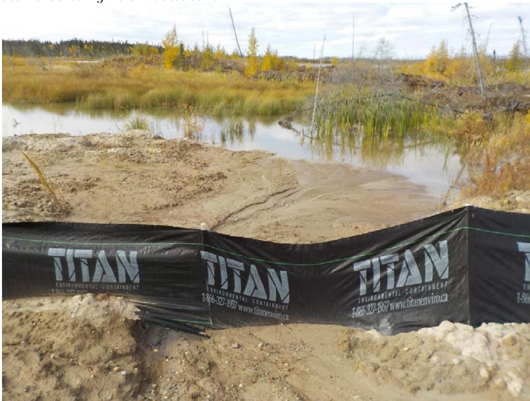
Sediment from EMPA D16 passing under a silt barrier and entering Wetland 51 buffer
