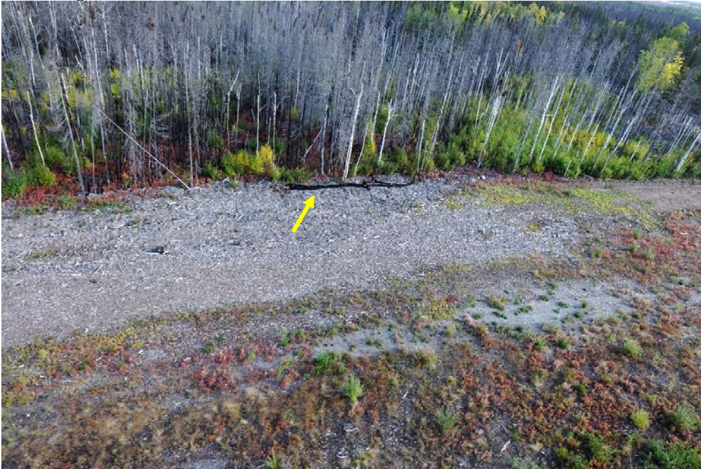
Silt fence installed at bottom of North Dyke slope near Wetland 45
