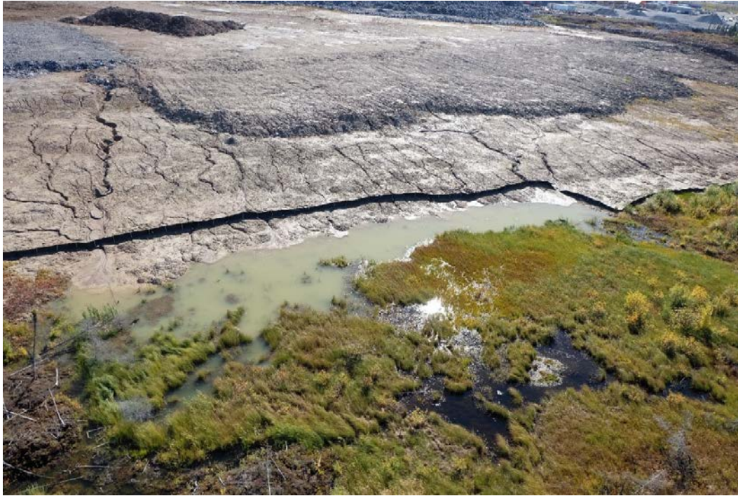
Aerial view of EMPA D16 slope near the east shore of Wetland 51, showing erosion channels and sediment entering marsh habitat buffer
