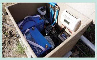
panels, batteries, and air compressors to force air bubbles through the water. The bubblers will be monitored to make sure that they are doing a good job and will be adjusted if necessary, so that fish swimming into Little Gull Lake will survive the winters.
