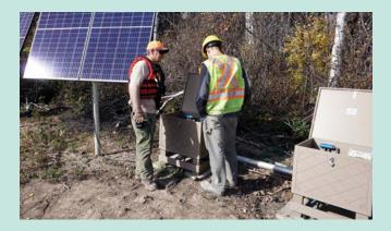
During the Keeyask environmental assessment it was identified that there would be a risk of fish trapped in the Little Gull Lake area dying during the winter due to low oxygen levels in the water. A solar powered system referred to as "bubblers", that add oxygen into the lake, was installed to protect the fish. The system uses solar
