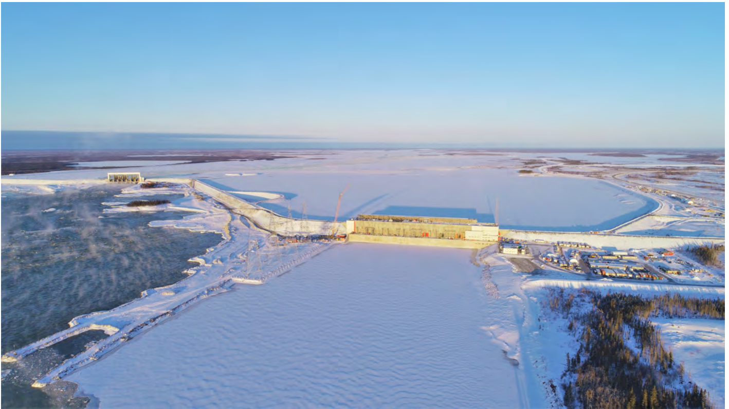
Keeyask tailrace and future reservoir area on Apr 6, 2020.
