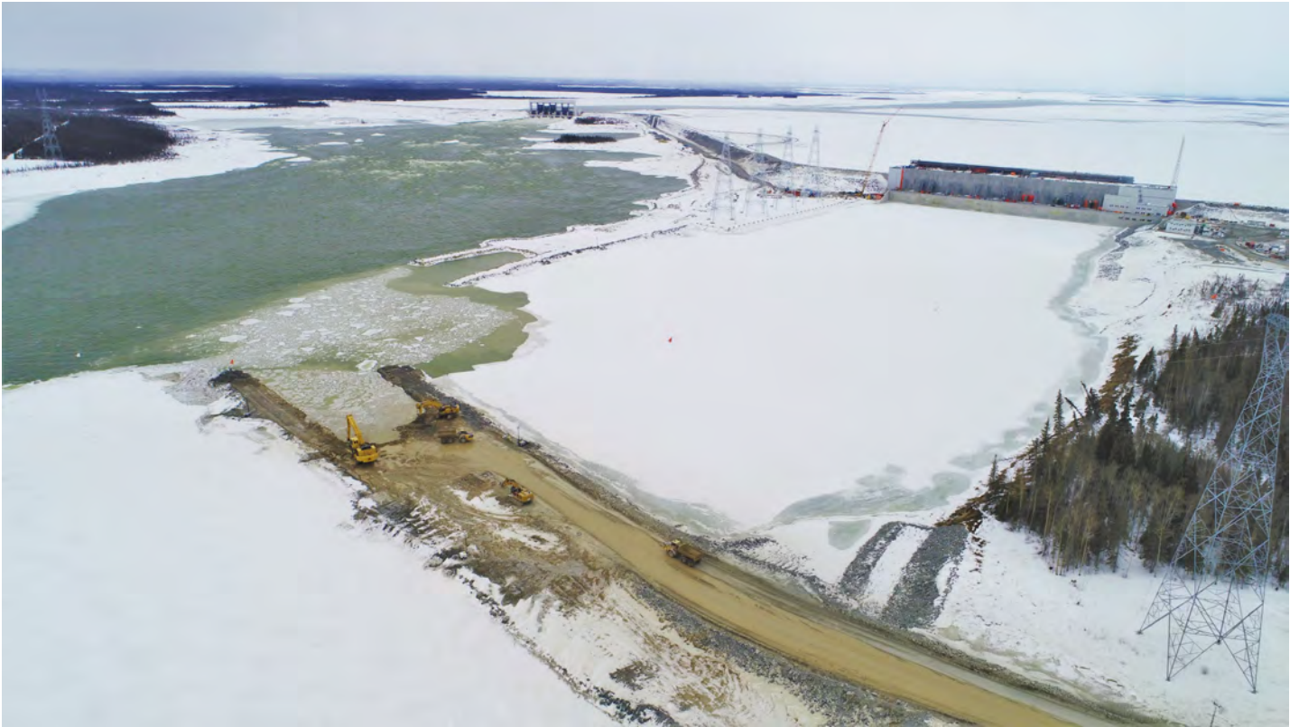
Tailrace cofferdam removal on April 15, 2020.
