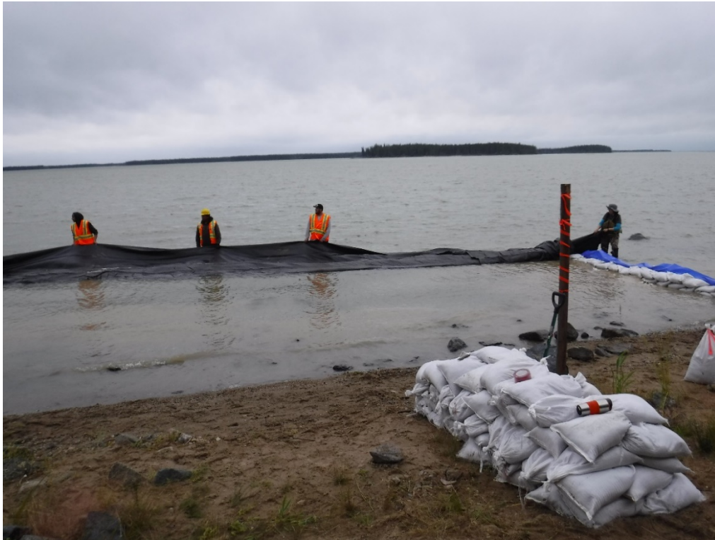
Photo 5: Setup of the aqua dam
