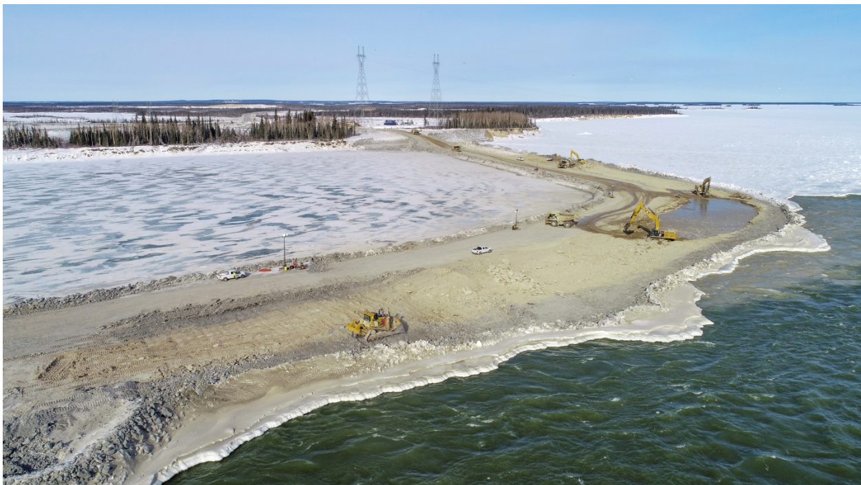
Figure 12: Removal in the wet of the TRCD. A small sediment plume can be seen on the right side of the photo. Photograph taken facing northeast, March 13, 2020
