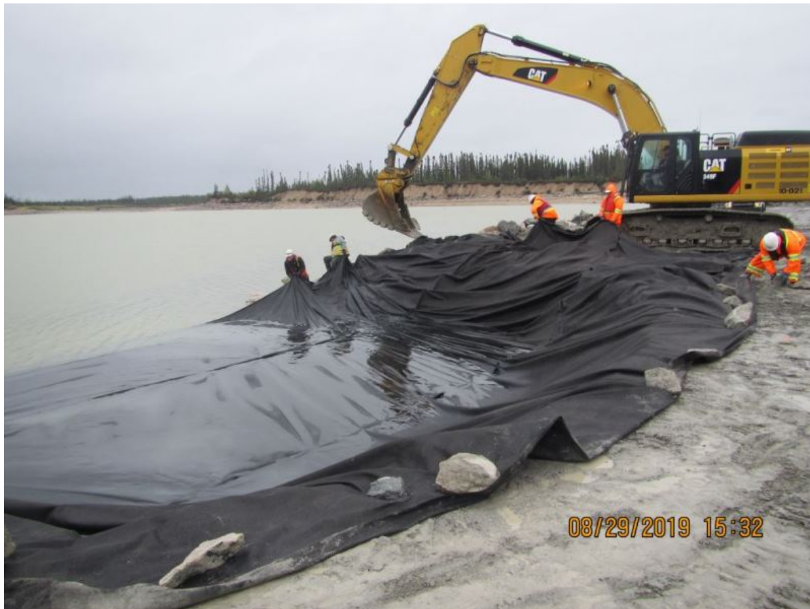
Figure 5: Geotextile is placed while constructing a finger drain at the South Dam
