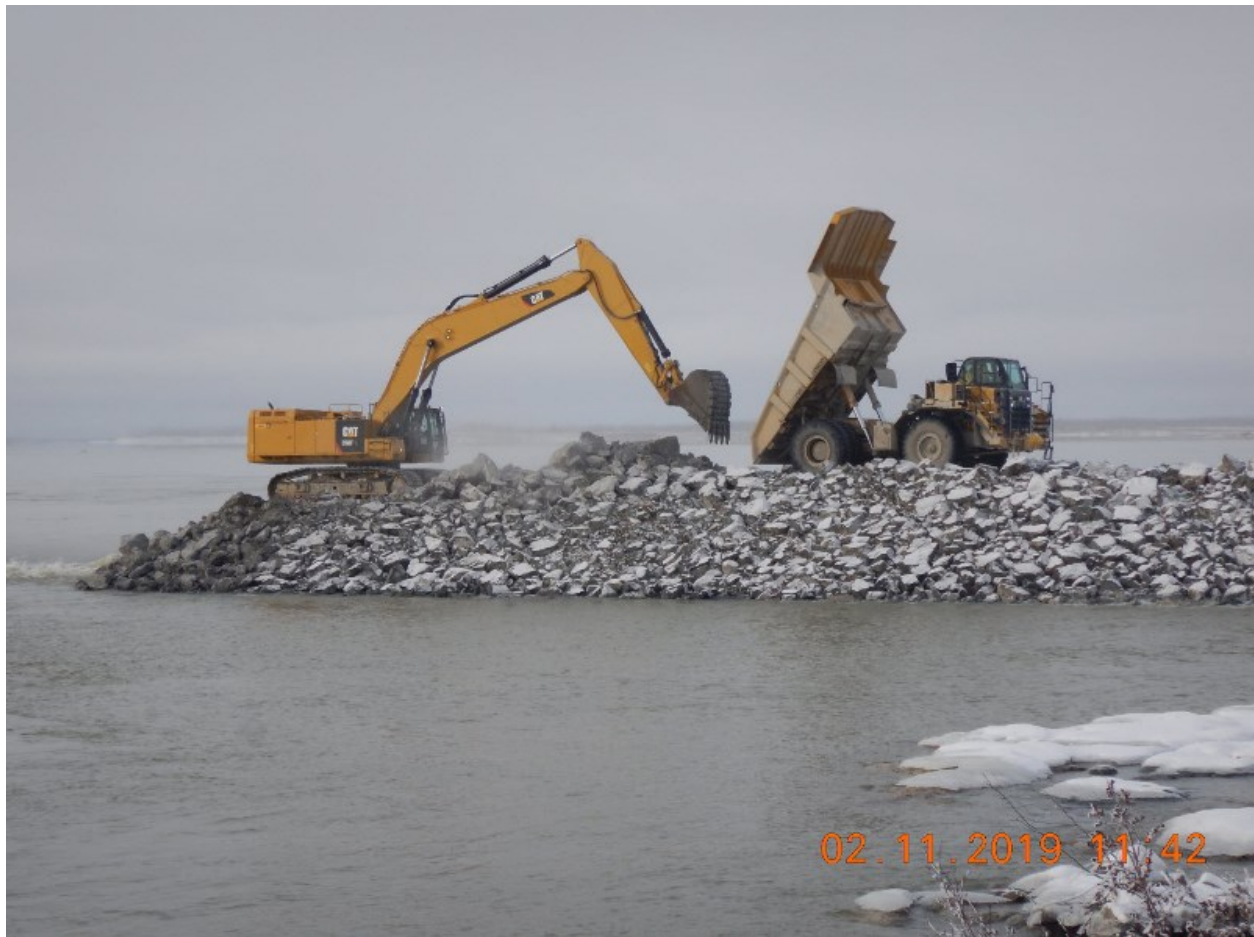
Figure 8: An excavator places large rockfill delivered by a haul truck into the river for the NCRG Extension
