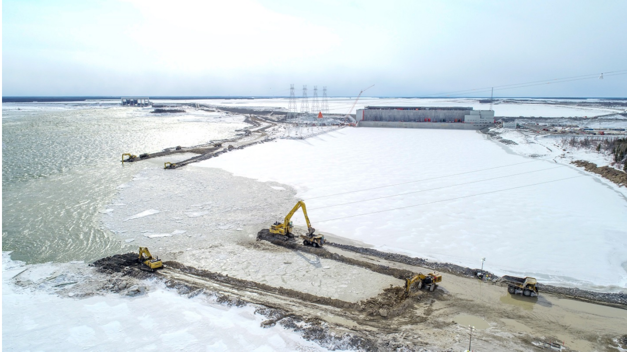
Figure 13: Removal of the TRCD facing west towards the Powerhouse. The inner and outer groins can be seen protruding past the core material, which was taken out first to minimize the suspension of the fine material. Photo taken on April 19, 2020.
