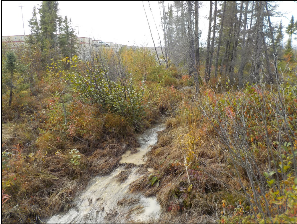
Photo 3-2: Channel created by running water from culvert northeast of Main Camp
