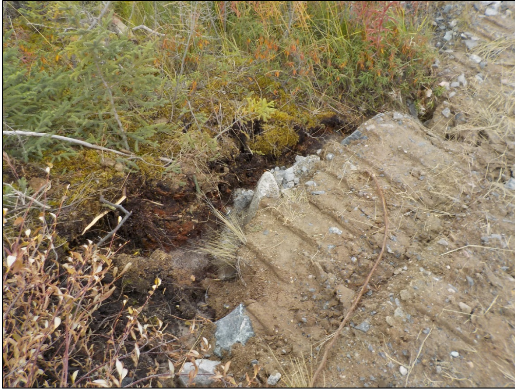
Photo 3-1: Erosion around fringes of excavated area adjacent to Borrow Area KM1
