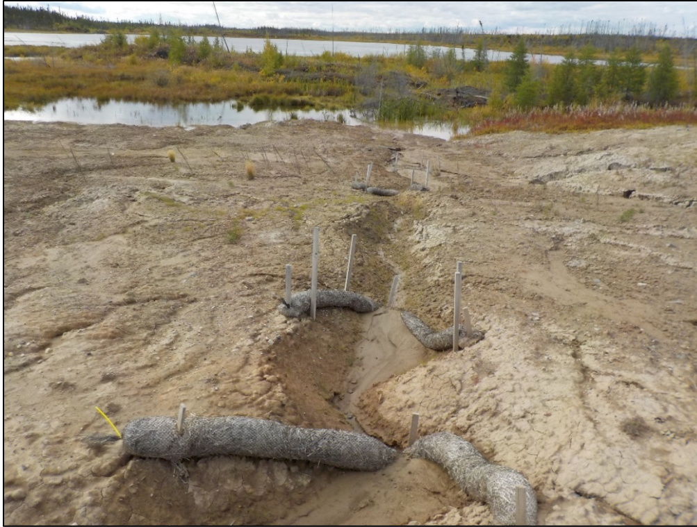
Photo 3-9: Straw wattles in gully along western edge of EMPA D16
