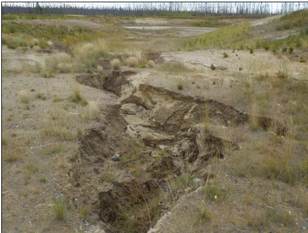
Photo 3-7: Erosion in Borrow Area KM1
