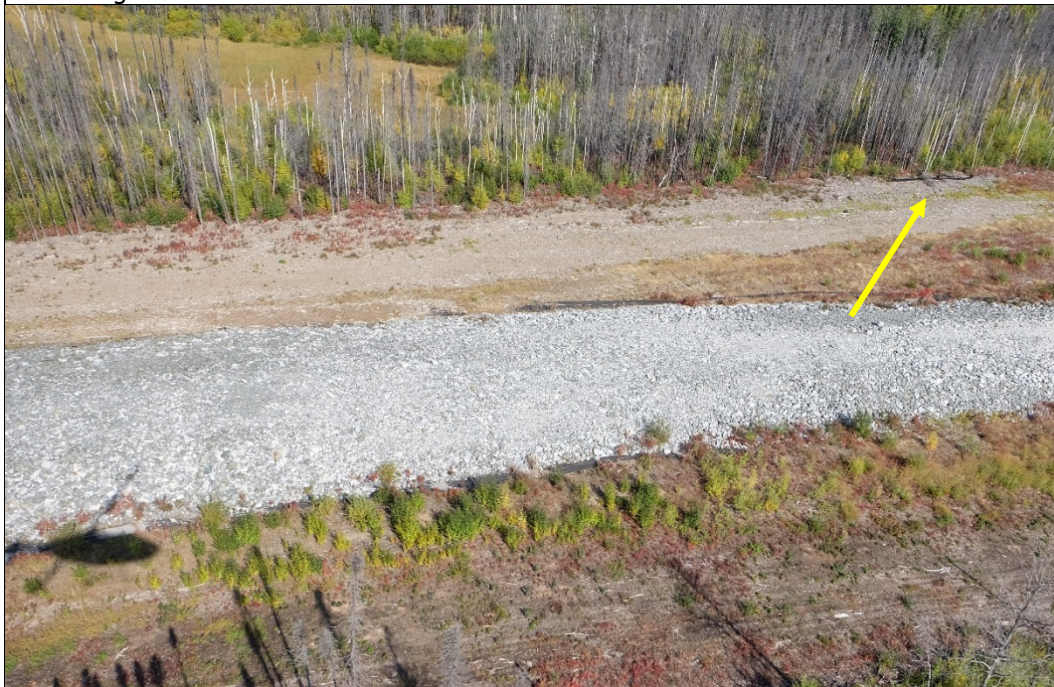
Silt fence installed at bottom of North Dyke slope near Wetland 45
