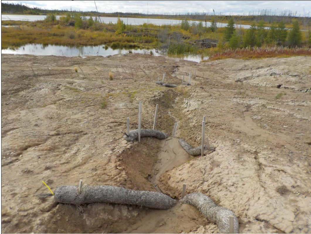
Sediment overtopping straw wattles placed within channels along western edge of Wetland 51
