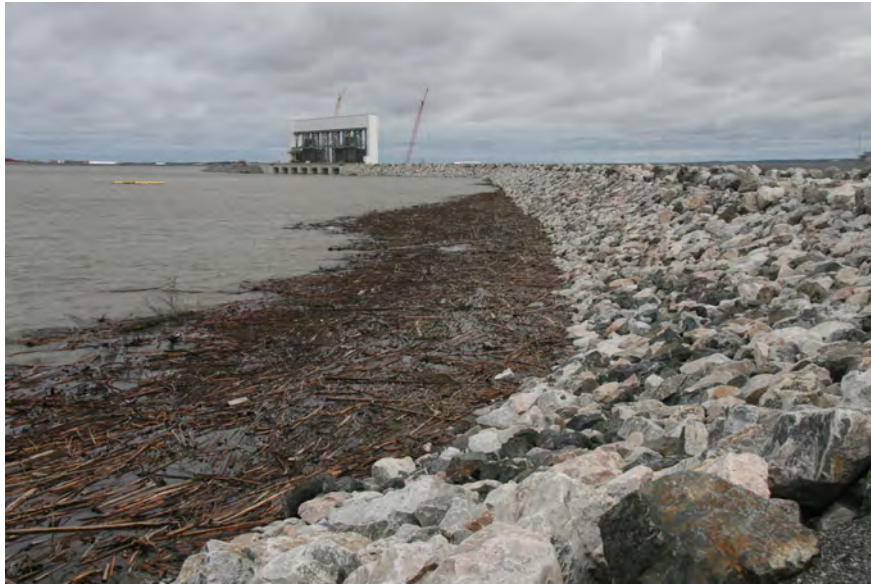
Keeyask Spillway and South Dyke with accumulating debris. Photo taken Sept 2, 2020
