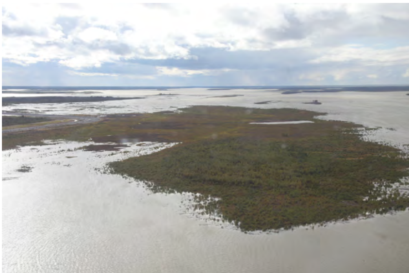
South Dyke looking west during impoundment.
