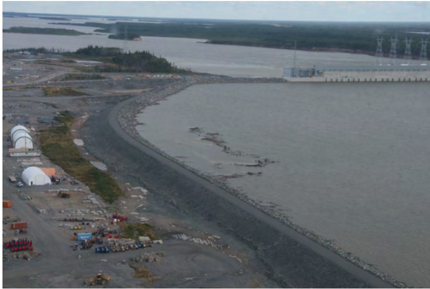
Keeyask Powerhouse and North Dyke. Photo taken Sept 1, 2020
