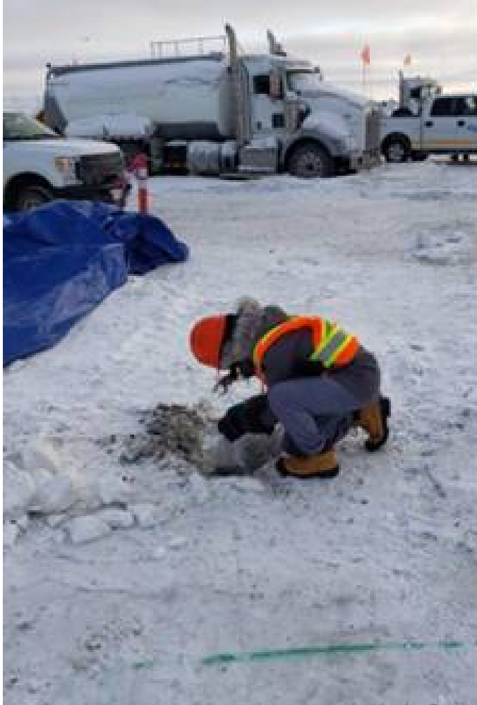
Photo 6: Youth Resource Coordinator digging up the ground after a diesel spill, remediation process
