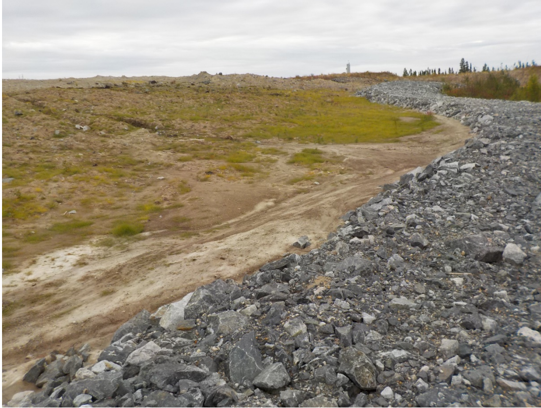
Photo 4-1: Well-performing portion of a rock berm at western end of EMPA D16
