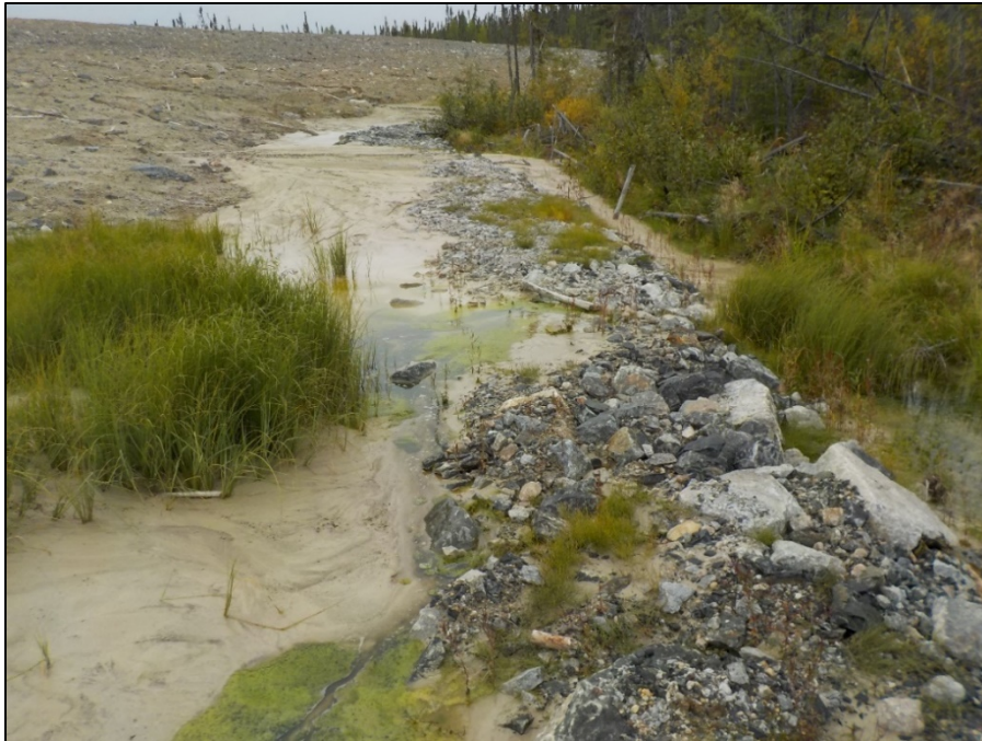
Photo 3-20: Sediment overtopping rock berms in EMPA D23(2)-E
