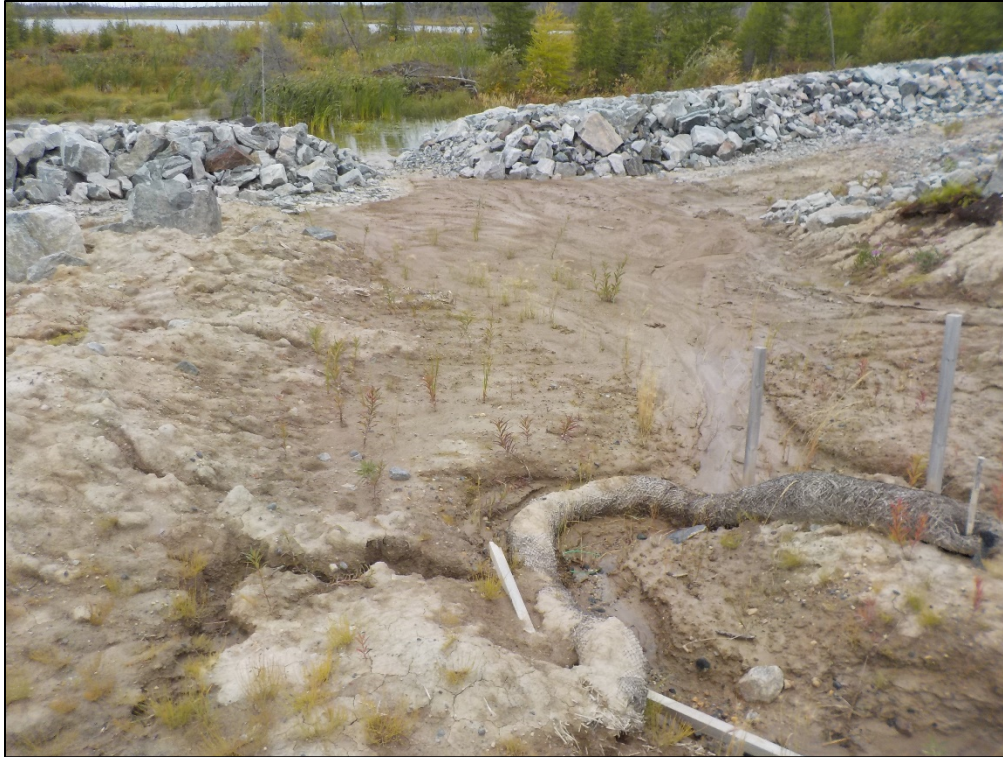
Photo 3-16: Sediment passing through straw wattles installed on western edge of EMPA D16
