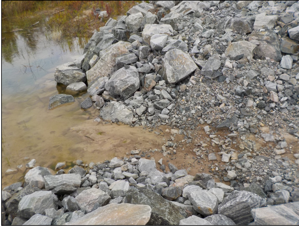
Photo 3-13: Gap in rock barrier in EMPA D16 that allowed sediment to pass through into adjacent marsh
