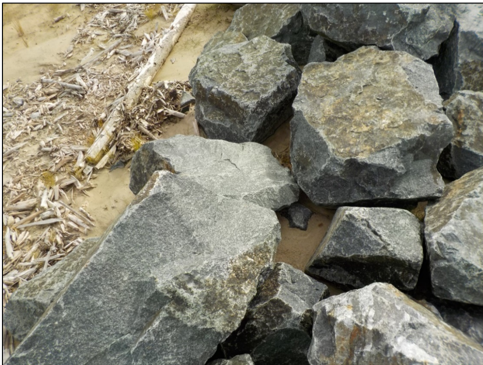
Photo 3-15: Rock barrier composed mainly of large boulders allowing sediment to pass through at the northern edge of EMPA D16
