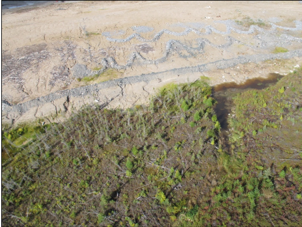
Photo 3-14: Rock barrier erosion at eastern edge of EMPA D16
