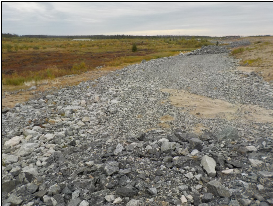
Photo 3-12: Low spot in rock barrier with sediment flowing over top at the northern edge of EMPA D16
