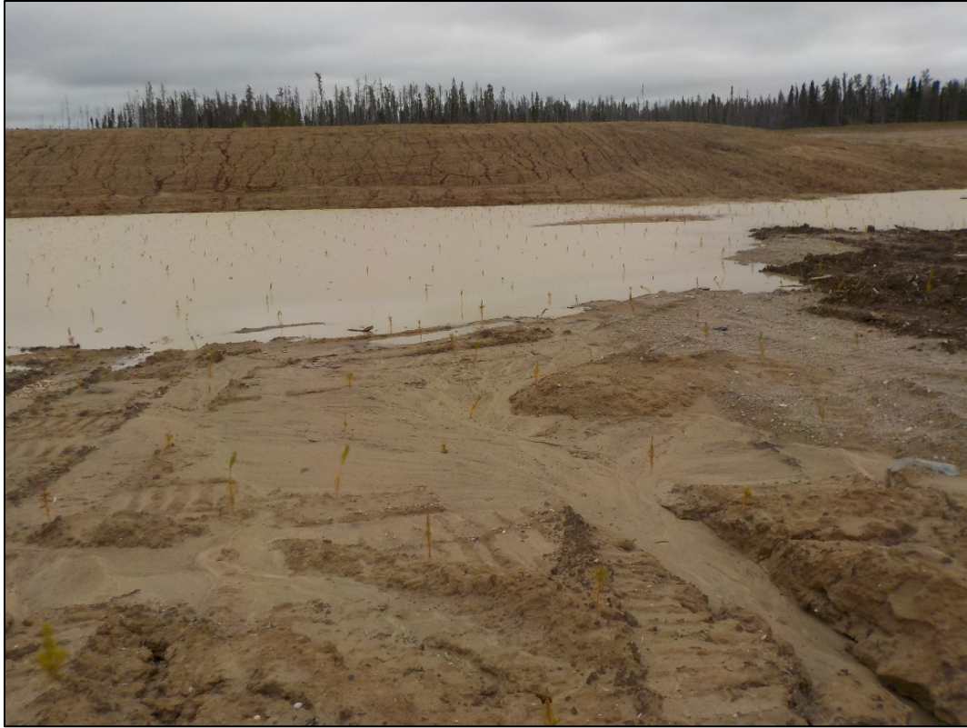
Photo 3-7: Erosion and ponded water affecting planted seedlings in Borrow Area G-3
