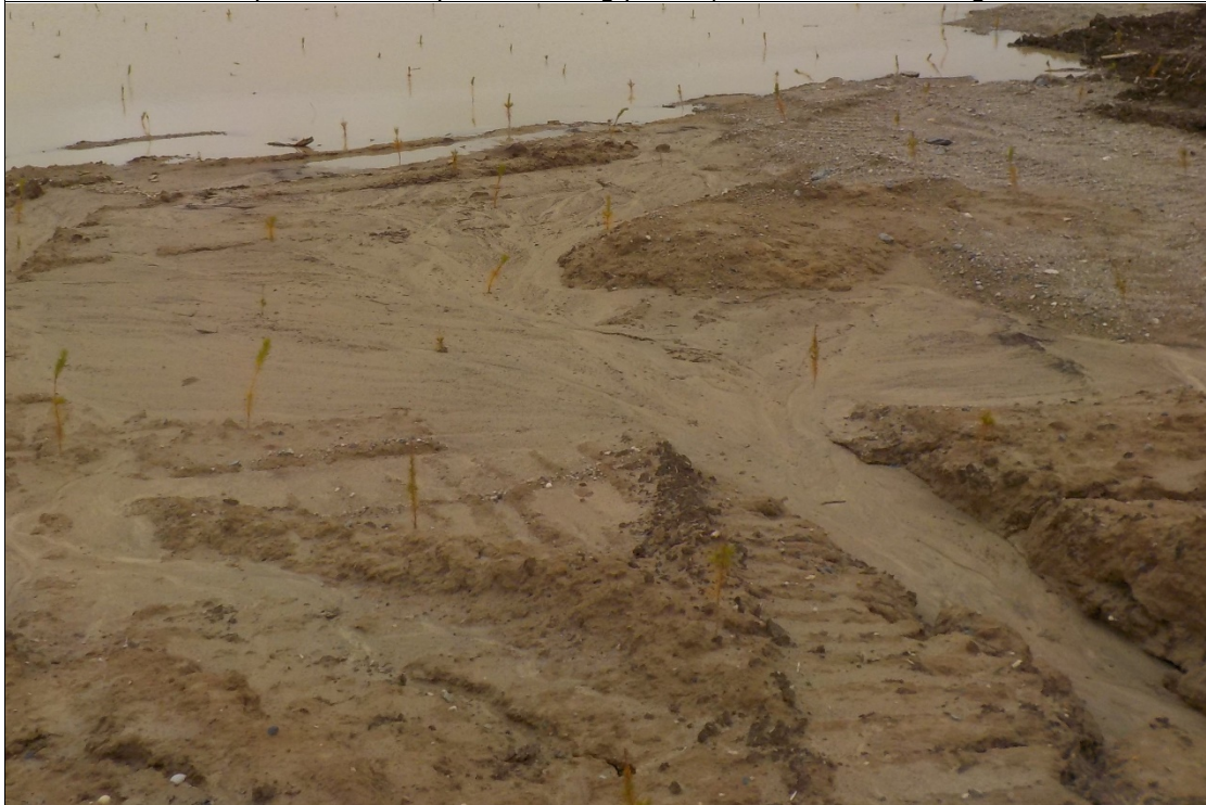
Example of erosion and water ponding in low areas, with seedlings washing away in same area
