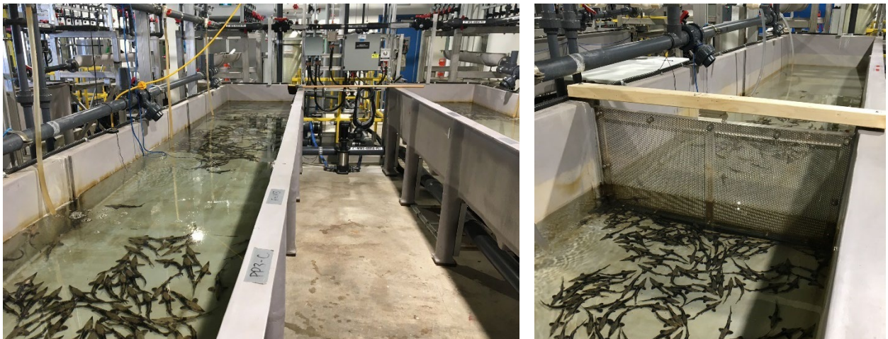
Photo 2: Rearing troughs in Pickerel Place used for interim Lake Sturgeon production. Installation of screens allow each tank to be divided into four sections.
