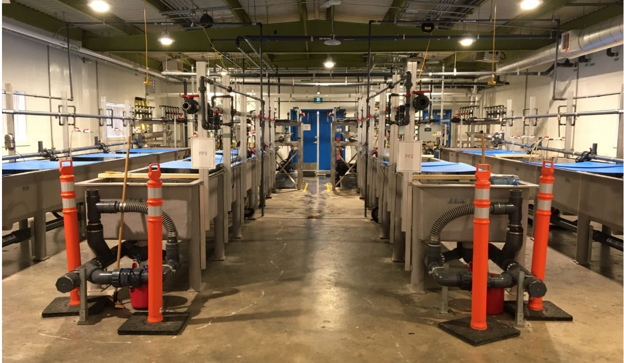
Photo 1: Water recirculating aquaculture systems in Pickerel Place. System 4000 is on the right and system 4100 is on the left.
