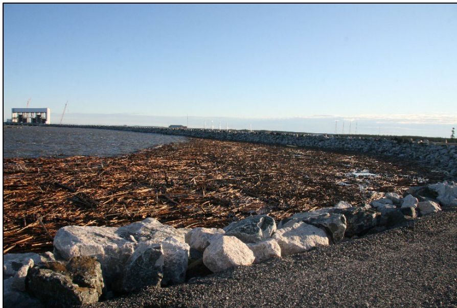
Woody Debris Adjacent to the South Dike
