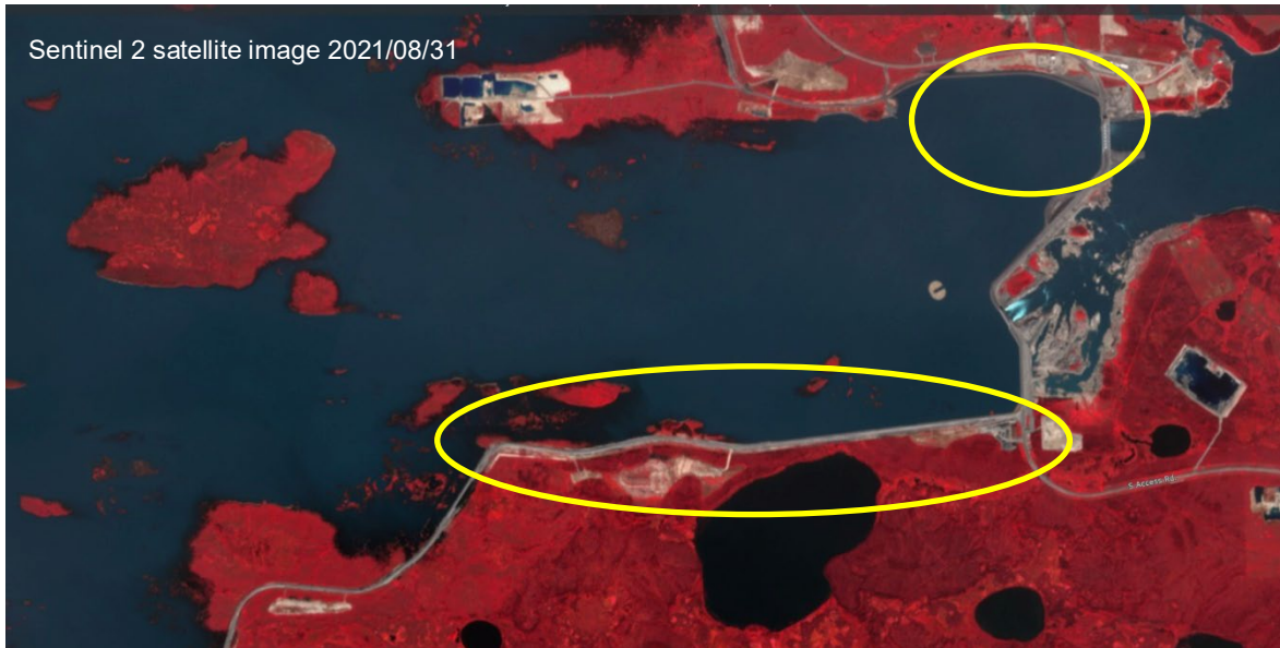
Figure 49: General work areas for work crew debris removal activities
