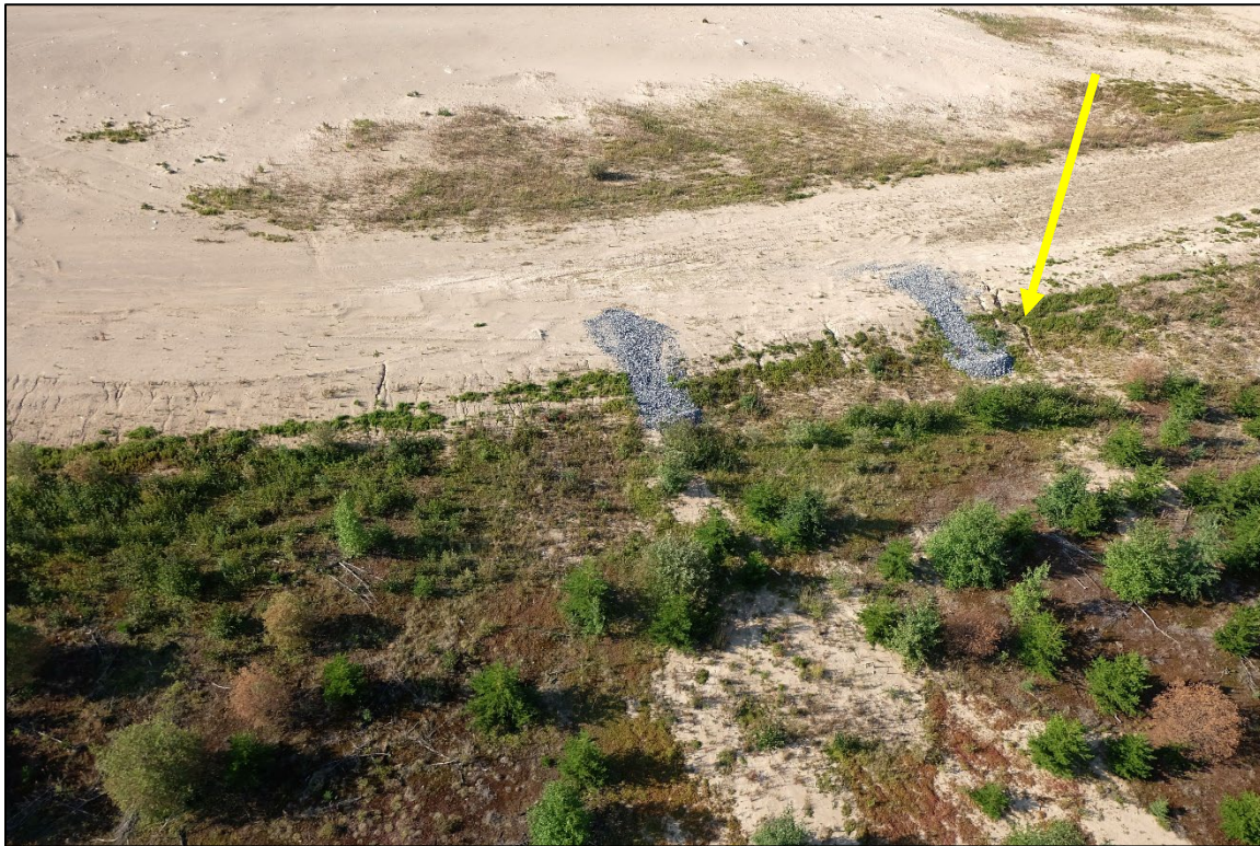
Photo 3-7: Rock placed in old erosion channels and new erosion channel (yellow arrow) at the northern edge of Borrow Area G-1 at KM 17 in 2022
