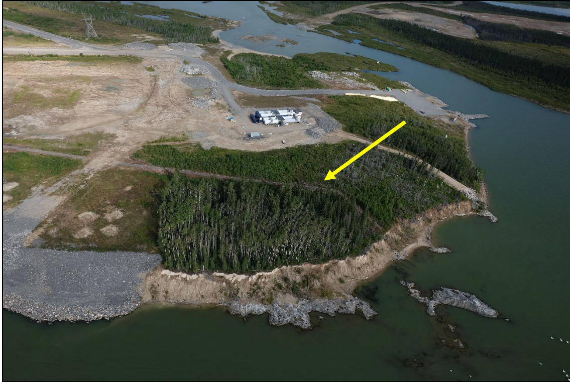
Photo 3-6: New clearing for safety fencing (yellow arrow) along the southern edge of Work Area C in 2022
