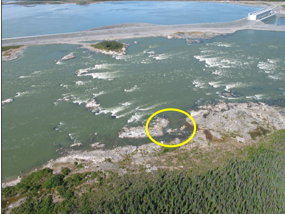
Photo 3-26: Portions of ice boom (yellow circle) washed up on the south shore of the Nelson River, downstream of the dam (dewatered area) in 2022
