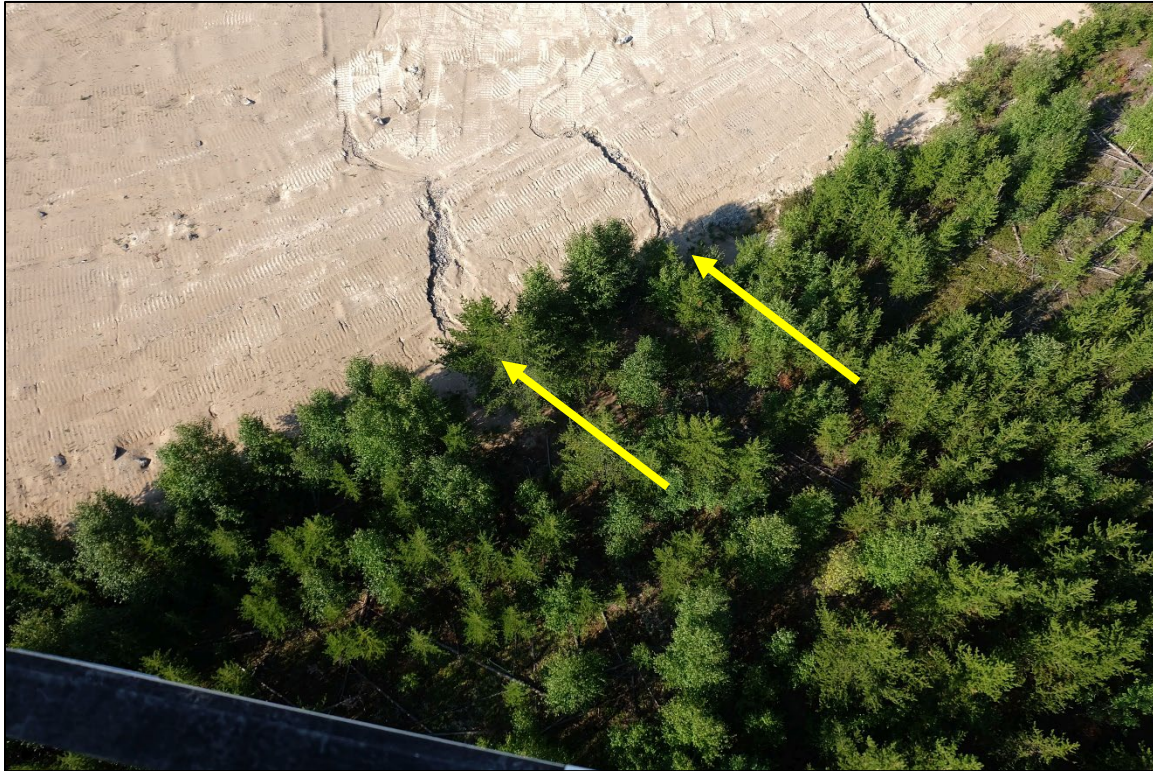
Photo 3-8: Erosion and sediment deposition (yellow arrows) on the northern edge of Borrow Area G-1 at KM 15 in 2022
