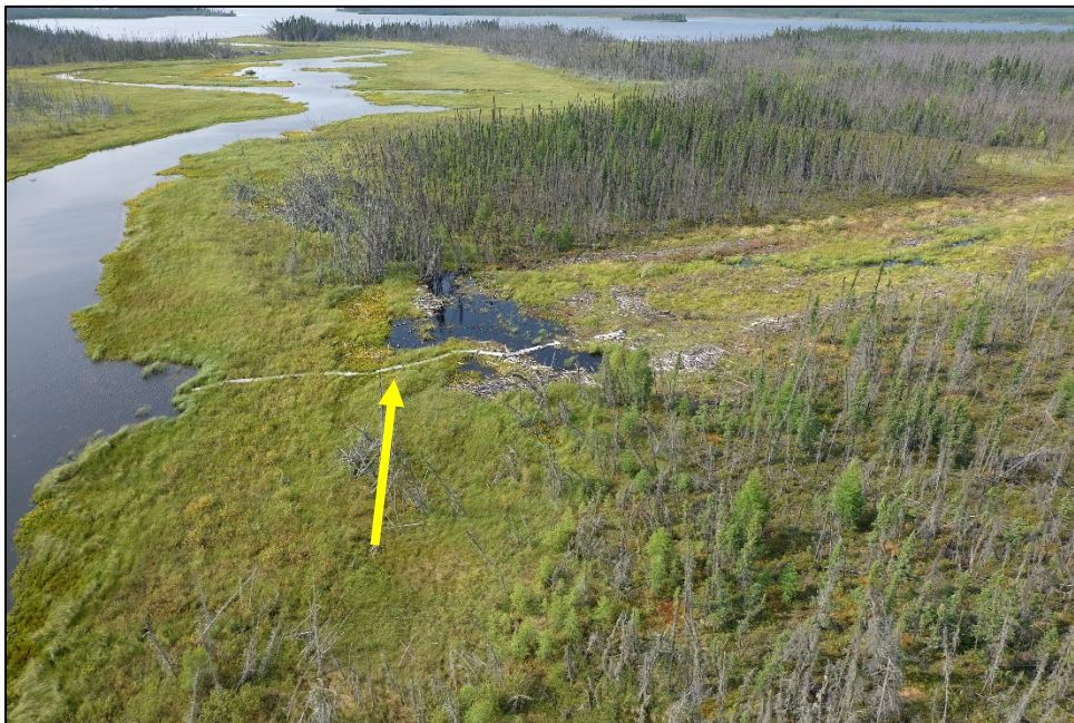
Photo 3-16: Plywood planks in Borrow Area E-1 access corridor in 2022
