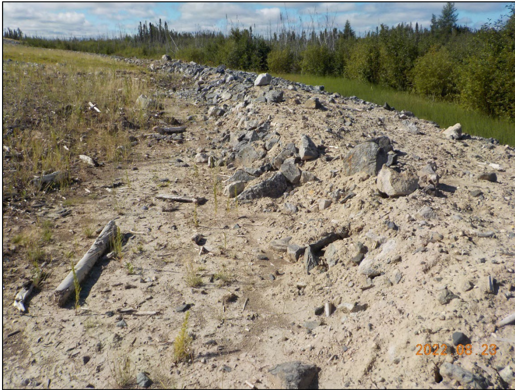
Photo 3-18: Reinforced rock berm in EMPA D16(1)-E in 2022
