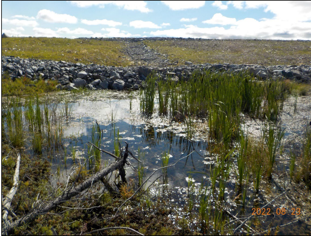
Photo 3-22: Filled-in gap in rock berm (center-top) adjacent to marsh (foreground) on western edge of EMPA D16(1)-E in 2022
