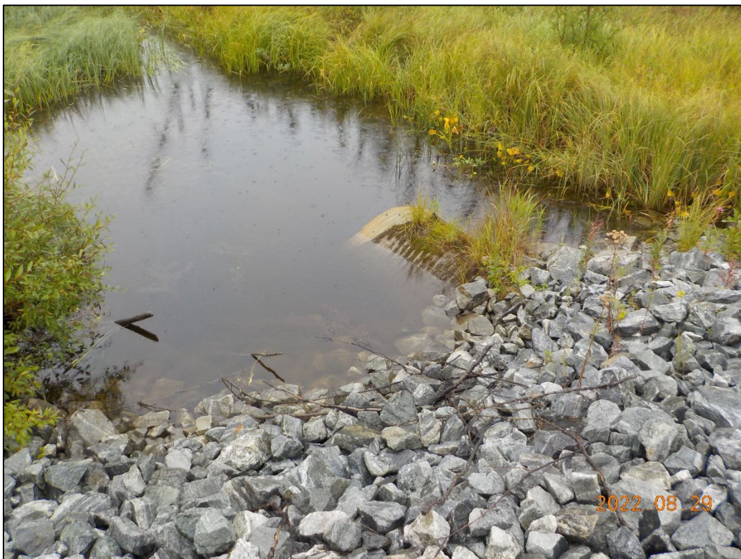
Photo 3-6: Culvert at the SAR in drainage channel at Wetland 57.
