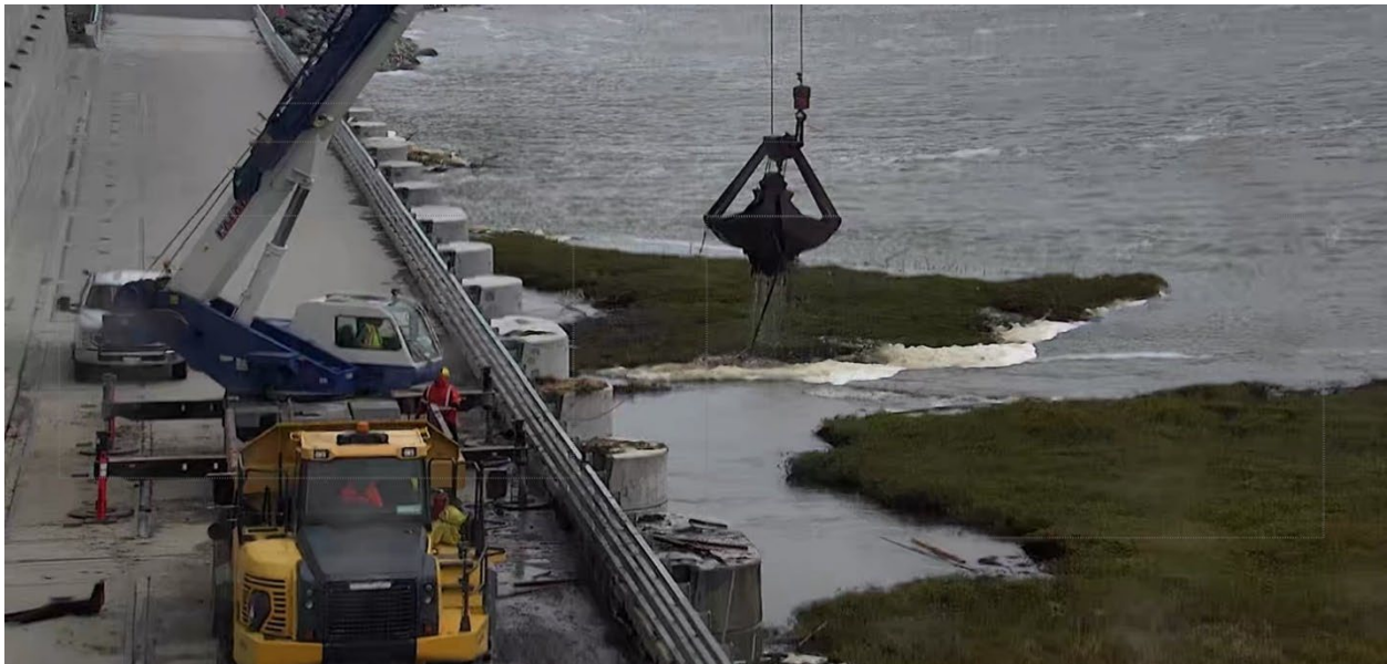
Photo 9: Crane with clam shell bucket on powerhouse deck removing peat island
